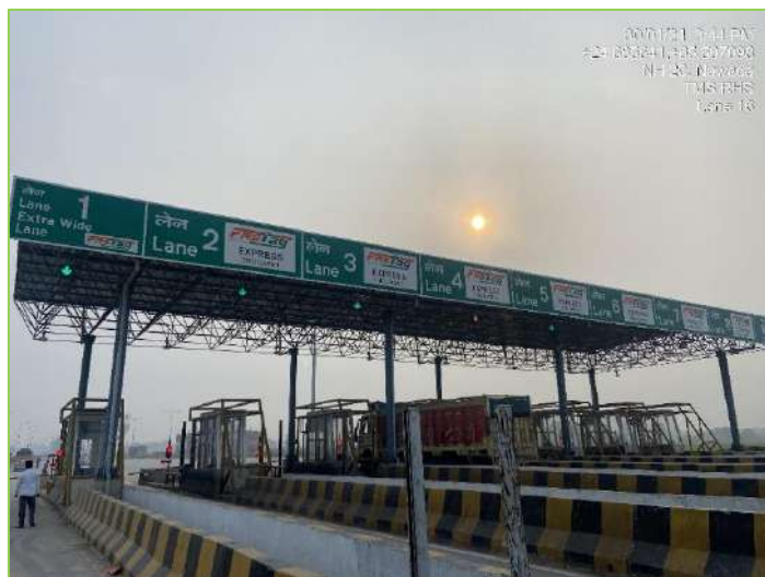
Figure 3-21: Over Head Lane Signal (OHLS).
