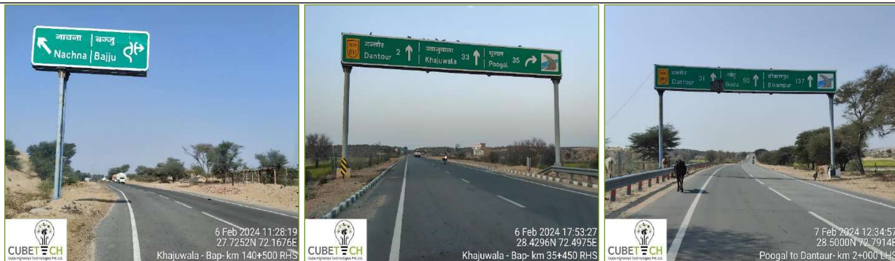
Figure 3-6: Overhead & Cantilever Gantry boards
