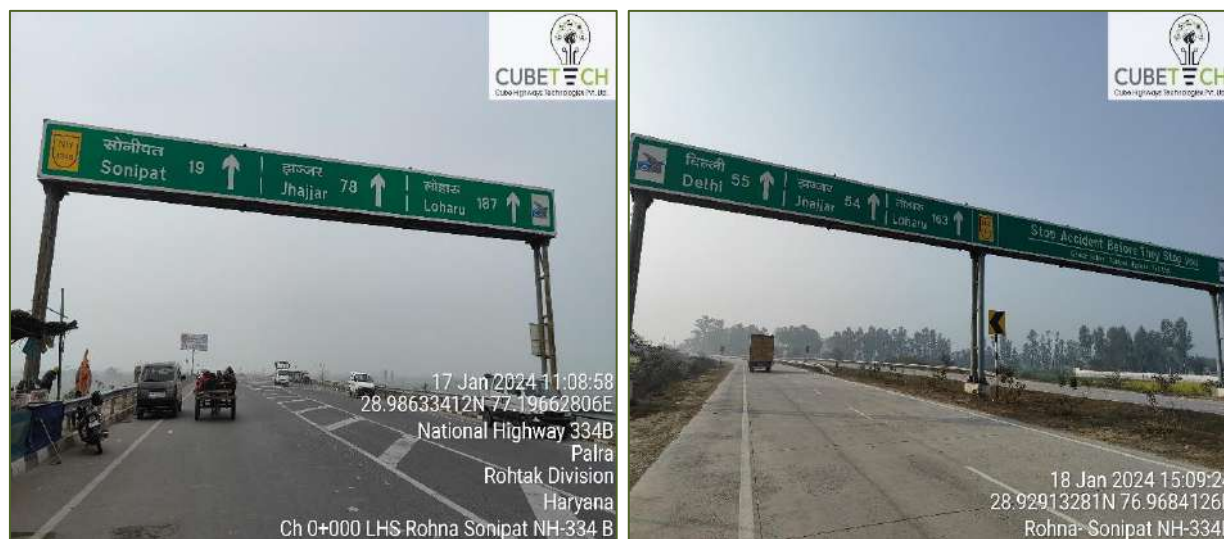
Figure 3-5: Overhead & Cantilever Gantry boards and VMS
