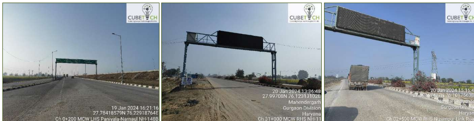
Figure 3-5: Overhead & Cantilever Gantry boards
