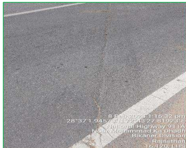
Figure: Transverse cracks
