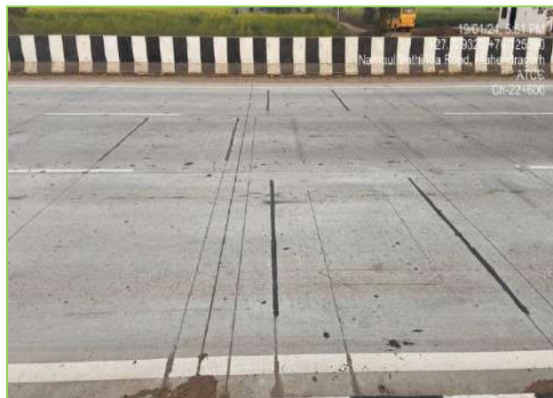
Figure 3-22: PLP Based ATCC.
