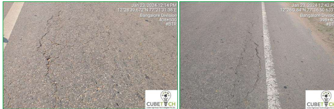
Figure 7-7: Alligator Cracks
