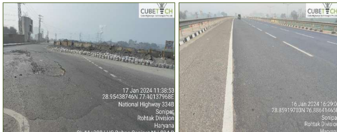
Figure: Alligator Cracks
