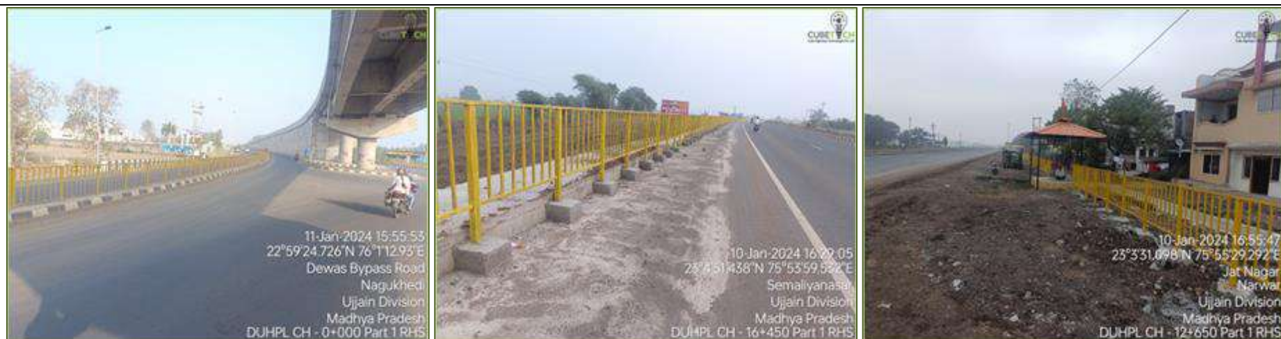
Figure 3-6: PGR along the project stretch
