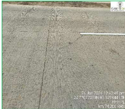
Figure: Corner Break
