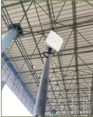
Figure 3-8: RFID reader.
