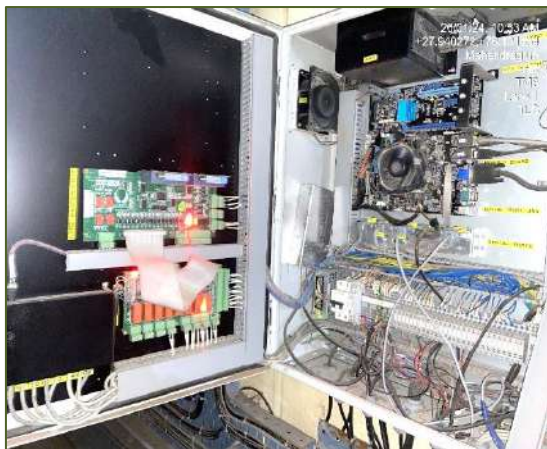
Figure 3-9: Toll Lane Controller inside Tunnel.
