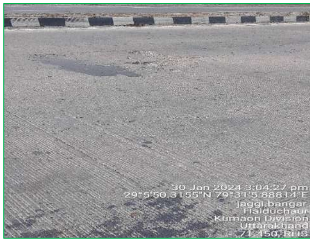
Figure: Scaling
