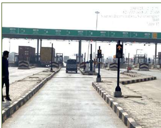
Figure 3-14: Over Head Lane Signal (OHLS).
