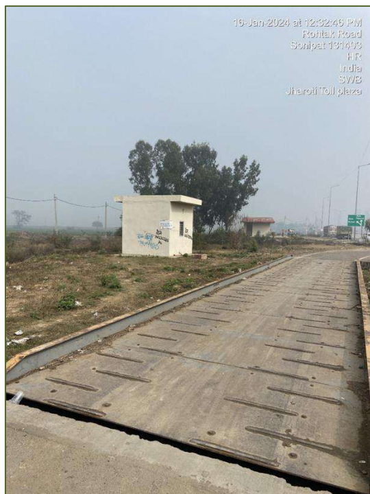
Figure 3-18: Static Weigh Bridge (SWB).
