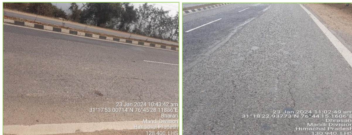
Figure: Alligator Cracks
