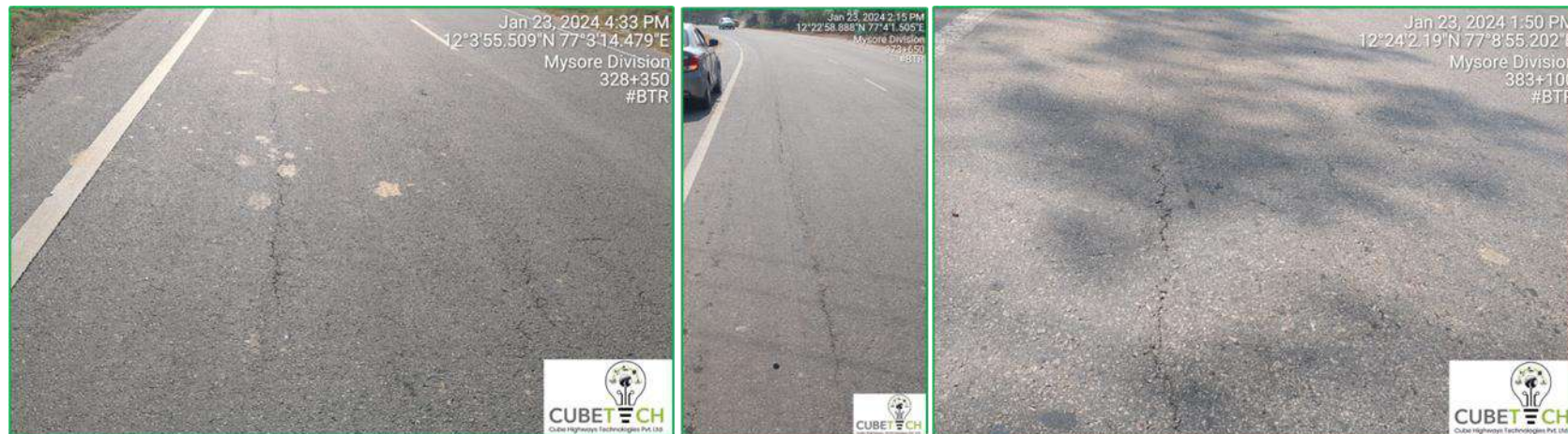
Figure 7-6: Longitudinal Cracks
