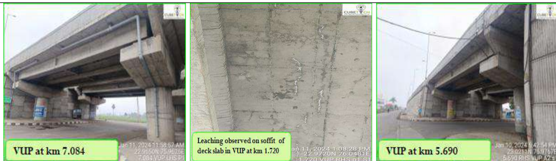
Figure 4-5: Condition of VUPs
