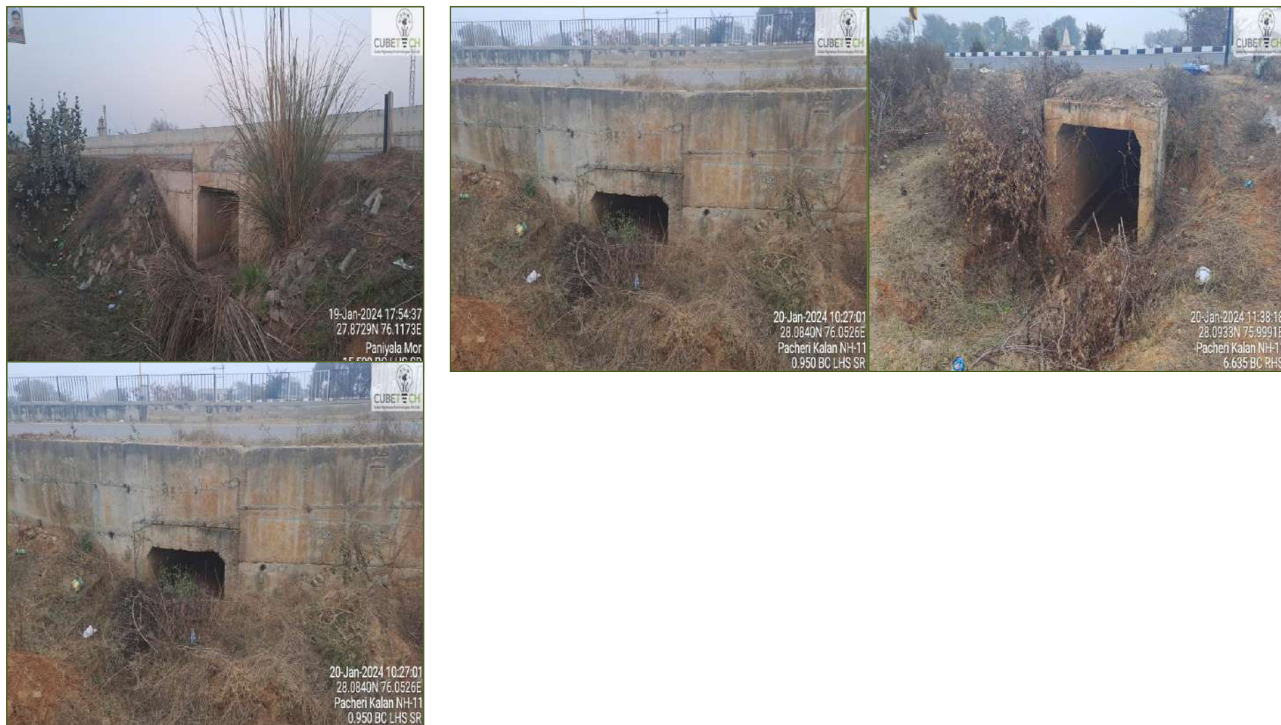
Figure 4-5: Condition of Culvert
