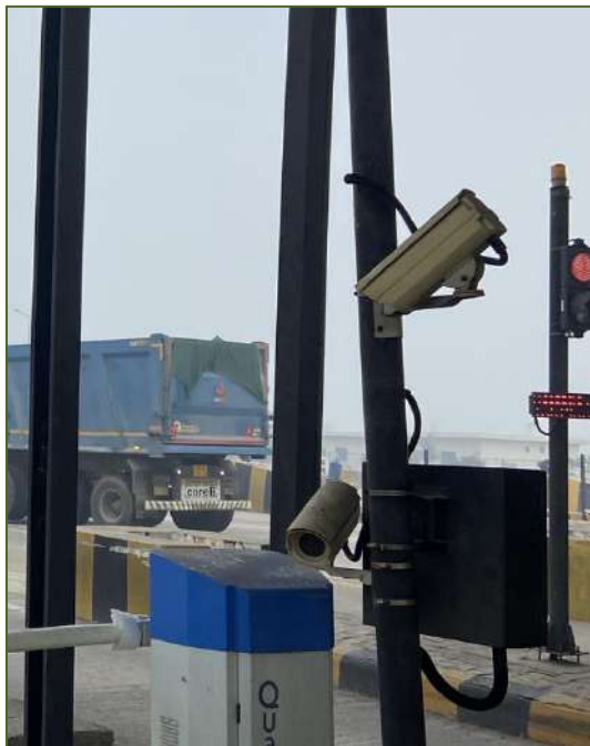
Figure 3-14: LPIC and ICS Cameras.
