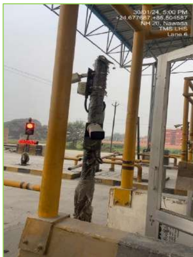
Figure 3-20: LPIC and ICS Cameras.
