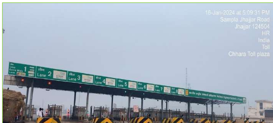
Figure 3-16: Over Head Lane Signal (OHLS).
