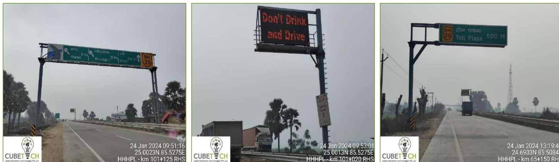
Figure 3-6: Overhead & Cantilever Gantry boards and VMS
