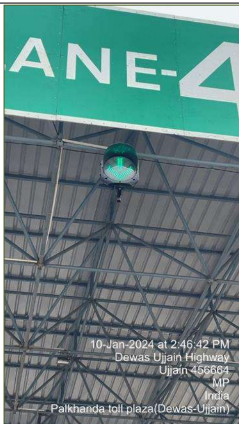
Figure 3-20: Over Head Lane Signal (OHLS)
