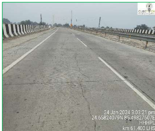
Figure: Longitudinal Cracks
