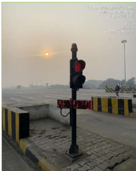
Figure 3-14: Traffic Light (TL) and User Fare Display (UFD).
