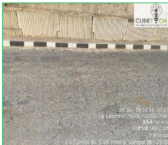
Figure: Alligator Cracks
