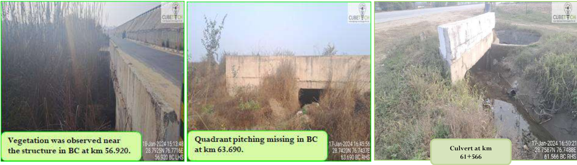
Figure 4-6: Condition of Culverts
