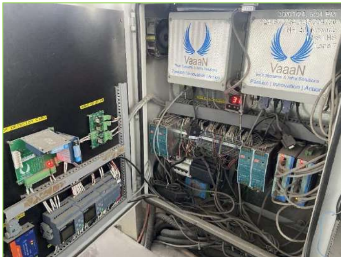
Figure 3-16: Toll Lane Controller inside Booth
