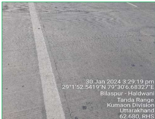
Figure 0-2: Tranverse Cracks
