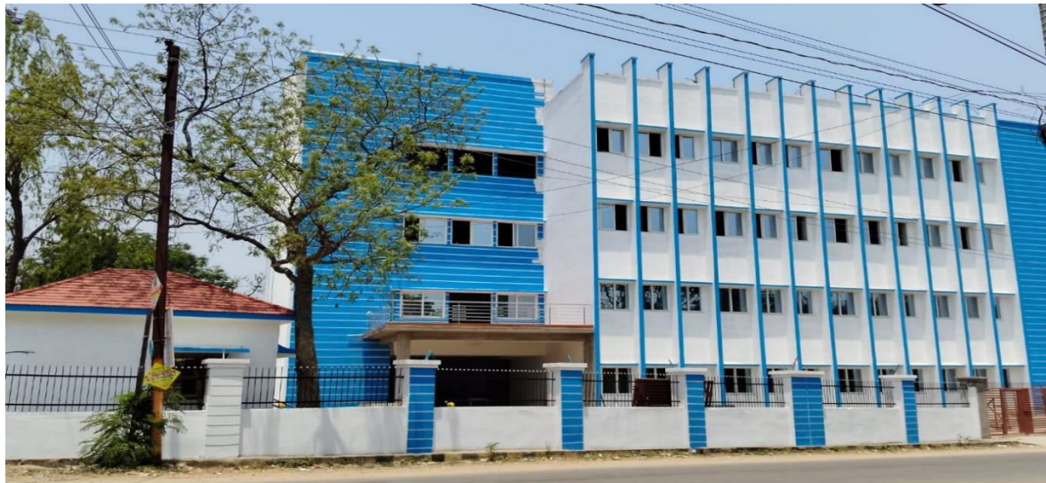
Construction of Commercial office
