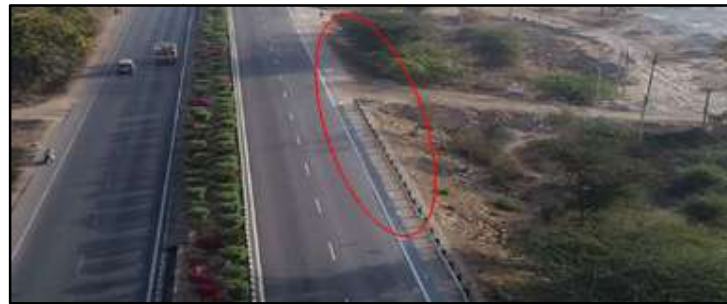
Figure 119. Photograph of deficiencies in safety barriers 627+900
