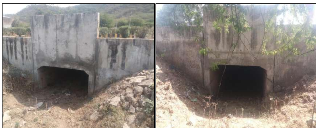
Figure 93. Photographs of box culverts 649/2 and 650/2 respect.
