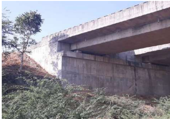
Picture-3: Toe wall observed
