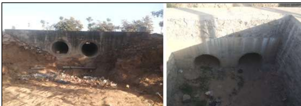
Figure 92. Photographs of pipe culverts 602/1 and 602/2 respect.
