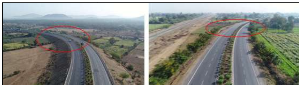
Figure 122. Photographs of deficiencies in curves delineation
