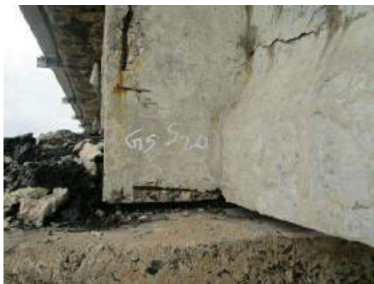
Pic - 7. 5 : Condition of Superstructure
