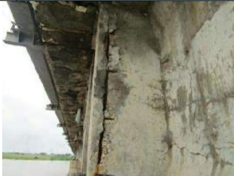
Pic - 7. 4 : Condition of Superstructure
