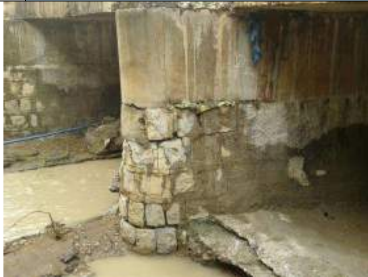
Pic - 6. 0 : Pier Damage Images
