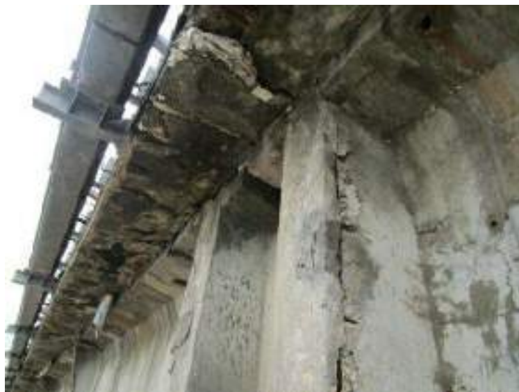
Pic - 7. 7 : Condition of Superstructure
