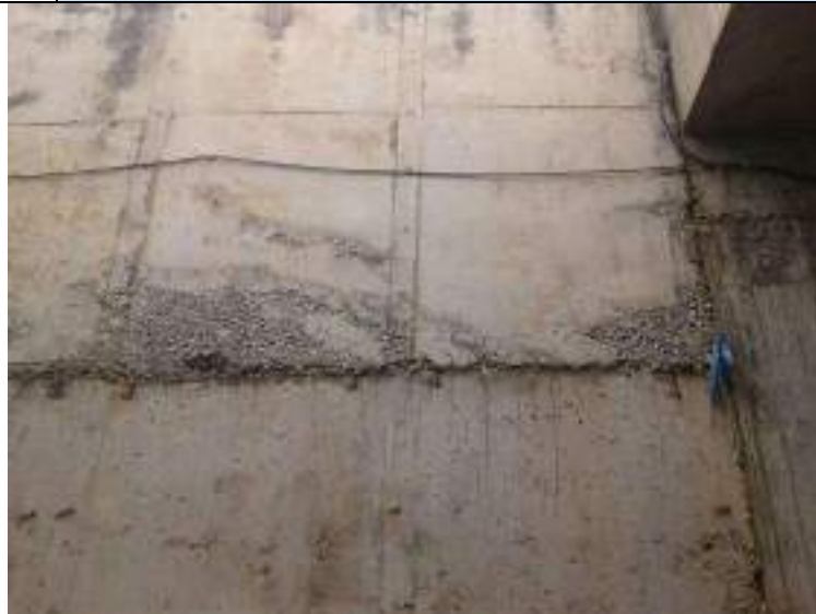
Pic - 5. 0 : Return Wall Damage Images
