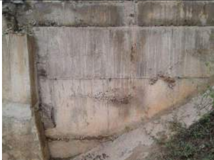
Pic - 6. 0 : Return Wall Damage Images
