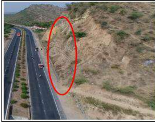
Figure 121. Photograph of deficiencies in safety barriers 647+800. Land/stone slide risk and impact
