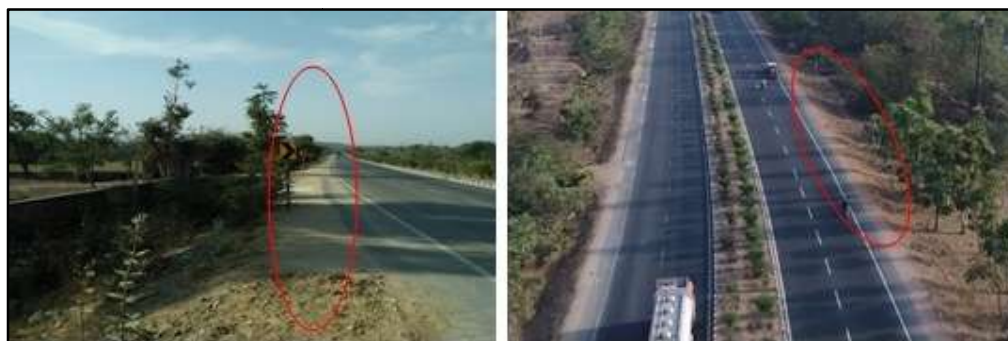
Figure118. Photographs of deficiencies in safety barriers 604+400 and 622+300
