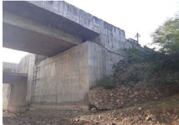
Picture-3: Side Protection Work
