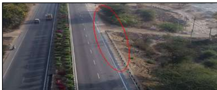
Figure 119. Photograph of deficiencies in safety barriers 627+900
