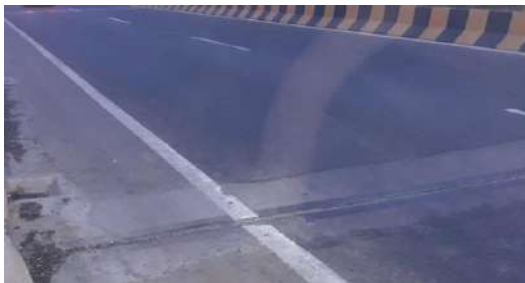
Picture-1: Expansion joint
