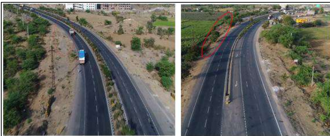
Figure 119. Photographs of deficiencies in safety barriers 659+800 and 659+600. Curve and elevated embankment
