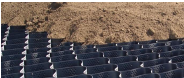
Erosion Control with Geocell
