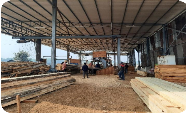
Sawn Timber Unit
