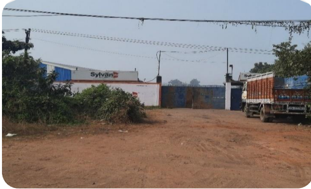
Main Gate (Entrance from NH-2)
