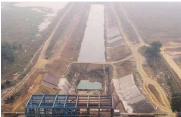
Construction of Check Dam and Water Pump House for Water Conservation, Forebay, Transition Zone and Intake channel, Internal Road & Drain etc, for CW and Make Up Water System
