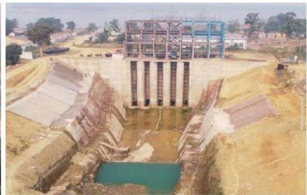
Construction of Check Dam and Water Pump House for Water Conservation, Forebay, Transition Zone and Intake channel, Internal Road & Drain etc, for CW and Make Up Water System
