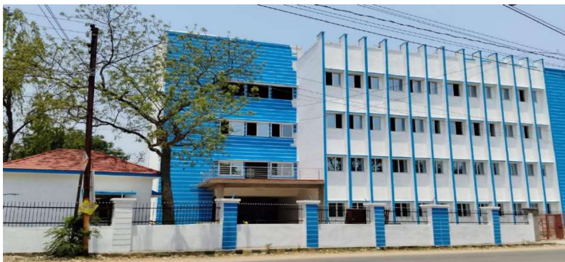
Construction of Commercial office
