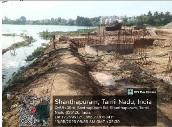
Design, Engineering, Build, operate and Commissioning of 12.51 MLD Capacity Sewage Treatment Plant at Santhapuram & 20.13 MLD Capacity Sewage Treatment Plant at Ramanaikken at Hosur
