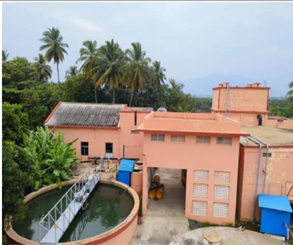
11 MLD & 3.15 MLD Water Treatment Plant at Gobichettipalayam
