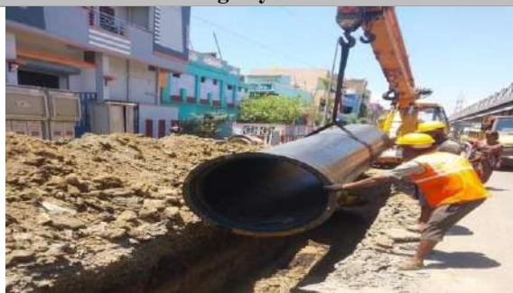
UGSS works at Tondiarpet, Chennai
