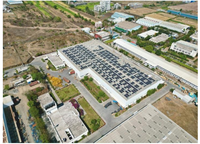
Chakan, Pune, Maharashtra - 750kWp
