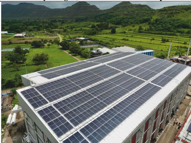
Satara, Maharashtra - 440 kWp
