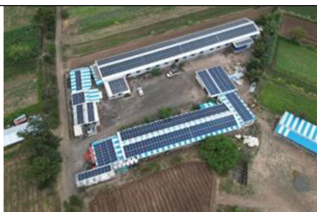
Satara, Maharashtra - 440kWp
