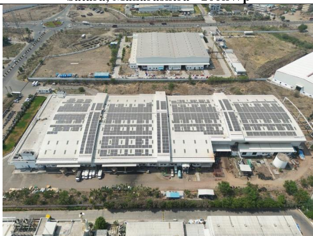
Chakan, Pune, Maharashtra - 1026kWp
