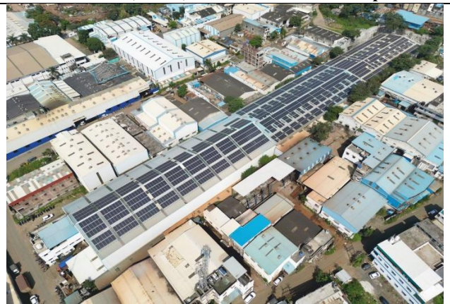
Chakan, Pune, Maharashtra - 1061kWp
