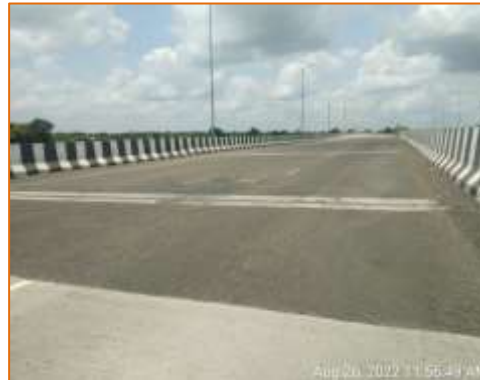
Flyover at km. 106.240 (LHS)
