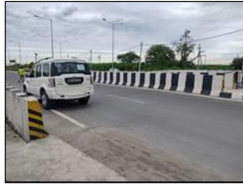
Minor Bridge at km. 77+613 (Top View)
