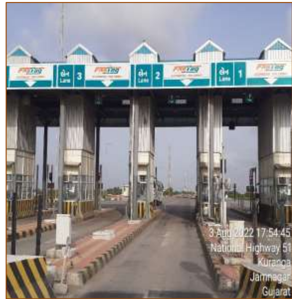
TP-2 at km. 470+875
