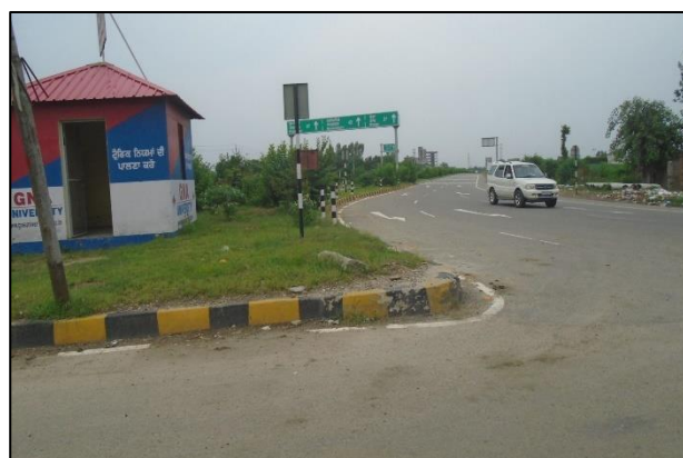
Start of Project Road - Right Carriageway
