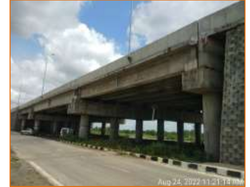
Side View of Flyover at km. 102.700 (LHS)
