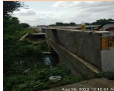
Box culvert at km. 133.524 - RHS (Reconstruction)
