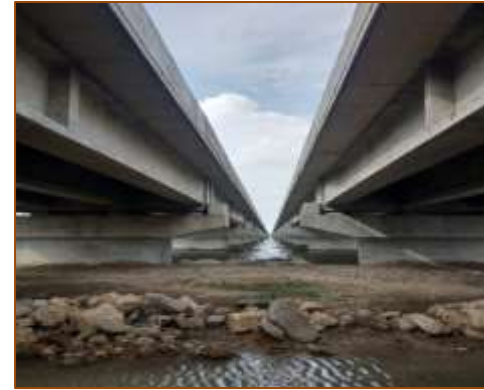
Mid Portion of MJB at km. 386+750
