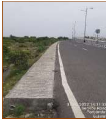
Built-up drain from km. 390+177 to km. 390+953 (RHS)
