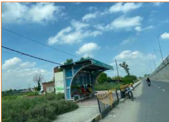
Bus Shelter at km. 775 + 900
