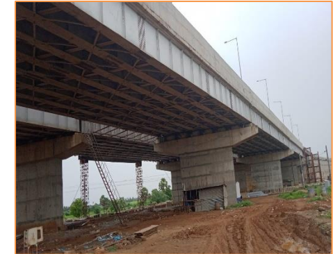
View of ROB at km. 18+677
