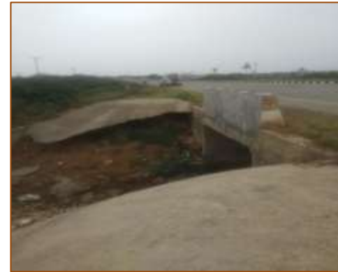
Slab culvert at km. 441+648 (LHS)
