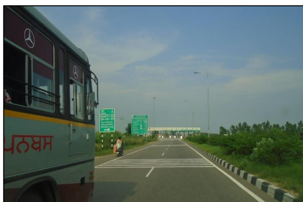
Behram Toll Plaza at km. 15+300
