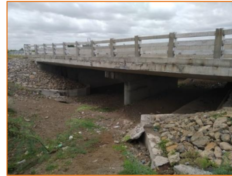
New Minor Bridge at km. 289.260
