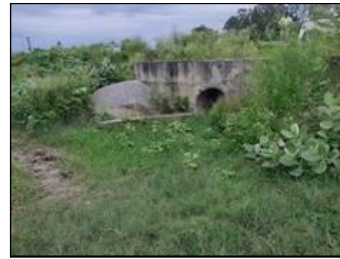
HP Culvert at km. 1+850
