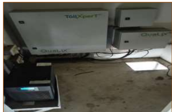
TP-2 at km. 470+875
