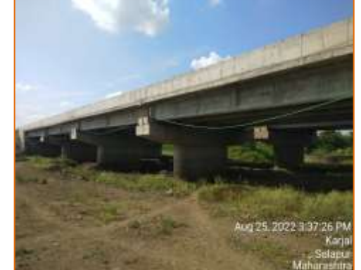
Side View of Major Bridge at km. 114.405 (LHS)
