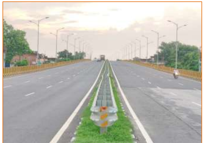
Highway Lighting at km. 740+300
