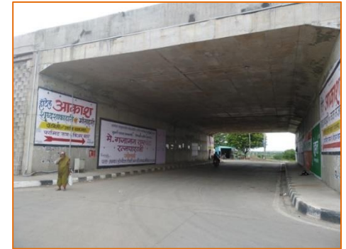
Light Vehicular Underpass at km. 283.650
