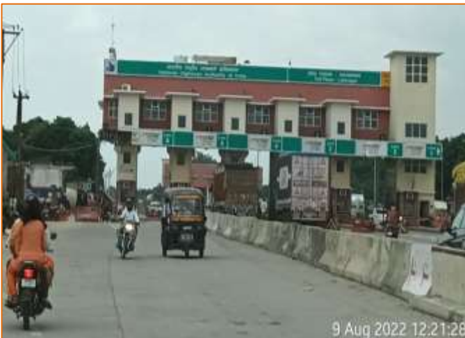
Toll Plaza including Admin Building at km. 747+581
