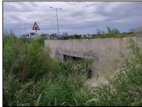
Box Culvert at km. 36+929
