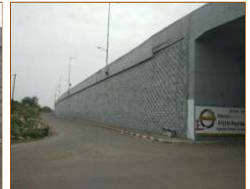
VUP at km. 396+865 (RHS) - A1 side
