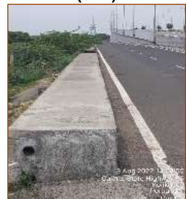
Built-up drain from km. 396+499 to km. 397+466 (RHS)
