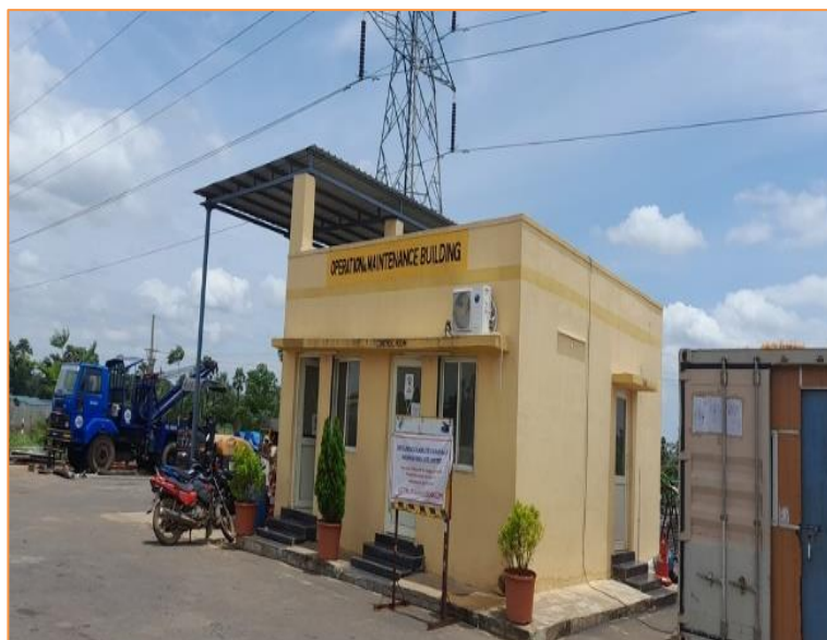
Figure 3-20 Operation and maintenance building at Toll Plaza
