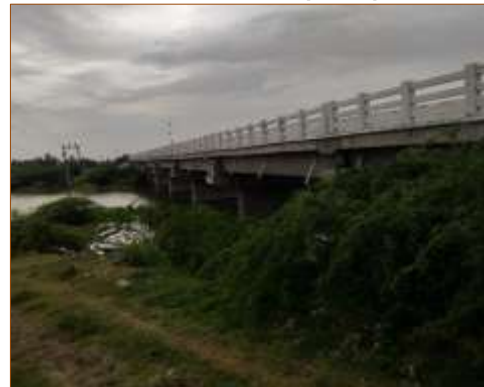
Side View of MJB - Widening at km. 420+180 (LHS)
