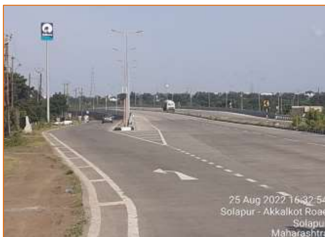
End of the Bypass at km. 106.526
