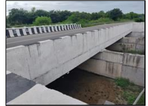
Minor Bridge at km. 72+900 (Top View)
