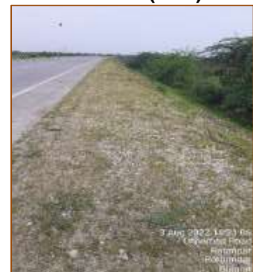
From km. 384+000 to km. 385+000 (RHS)
