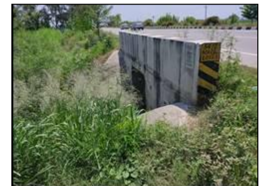
Box Culvert at km. 53+510
