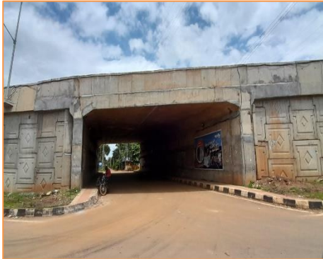
View of LVUP at km 27+790
