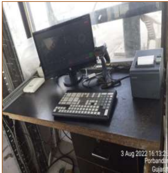
TP-1 at km. 409+500
