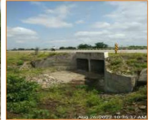
Box culvert at km. 126.643 - LHS (Reconstruction)
