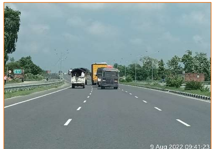
Road Marking at km. 761+200.
