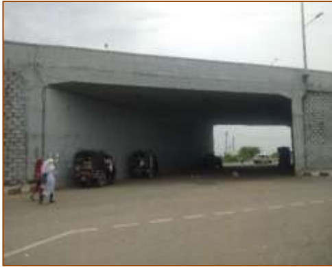
VUP at km. 432+050 (LHS) - Skew (Miyani) under COS
