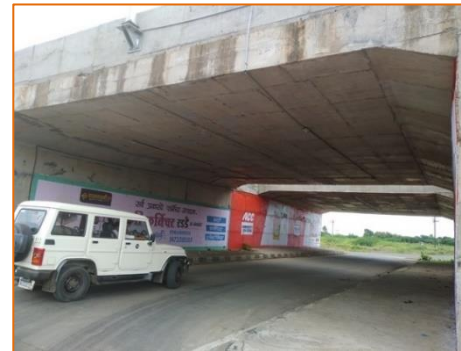
Light Vehicular Underpass at km. 320.900
