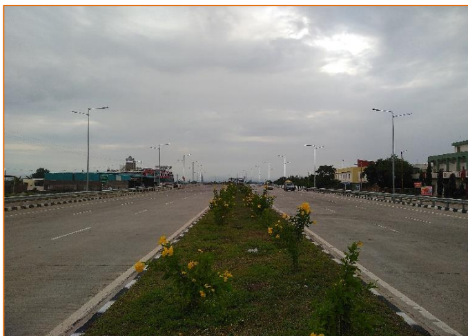
Pavement Condition at km. 285+750 (BHS)
