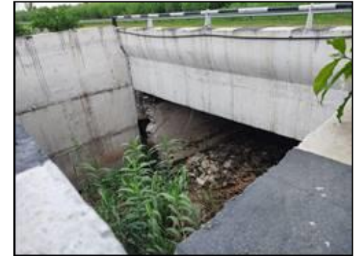
Minor Bridge at km. 76+815 (Structure View)
