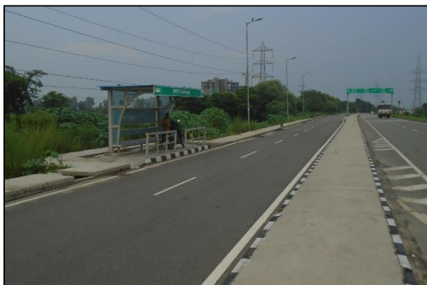
Bus Bay at km. 0+740
