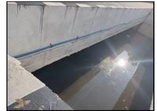
Minor Bridge at km. 71+727 (Structure View)
