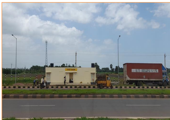
Truck Lay bye at km. 16+520
