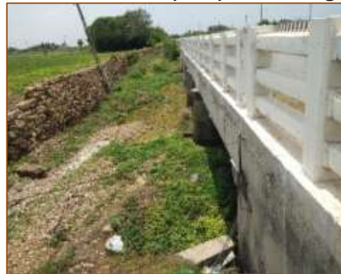
Side View of Minor Bridge at km. 440+350 (RHS) - Widening
