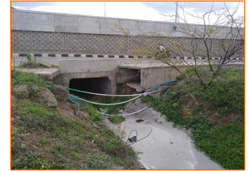
Box Culvert at km. 285+300
