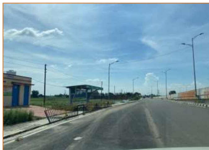
Toilet Block at km. 775+910
