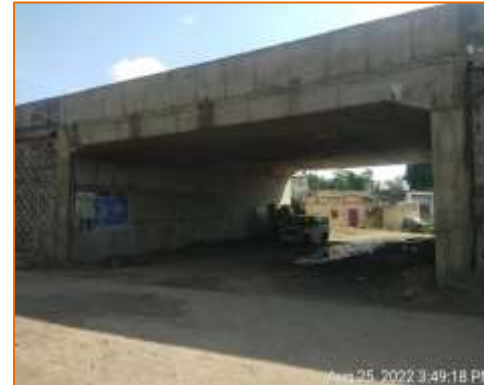
Side view of LVUP at km. 114.080 (RHS)
