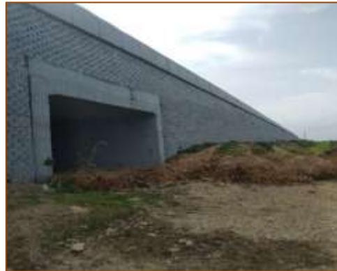
VUP at km. 393+695 (RHS)
