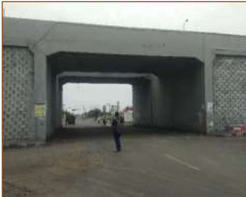
VUP at km. 400+681 (RHS)
