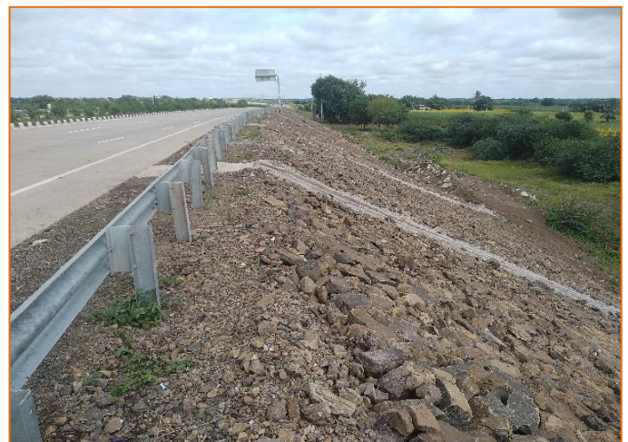
Slope Protection work at km. 298+300
