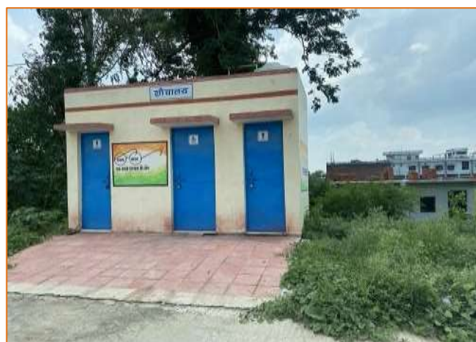
Toilet Block at km. 768+420
