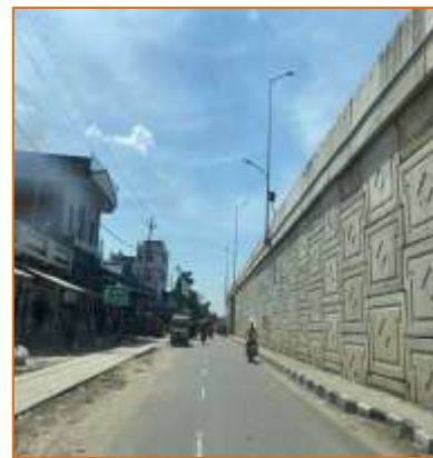
Service Road at km. 734+175
