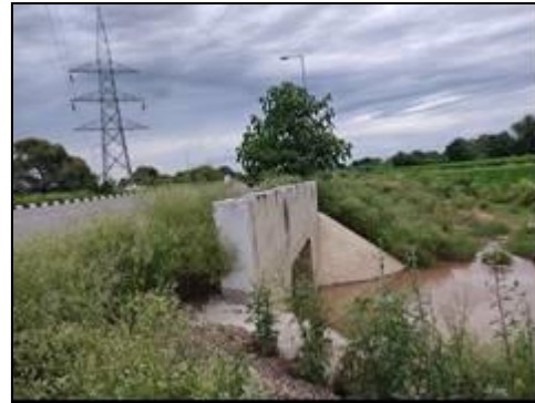
Box Culvert at km. 17+946
