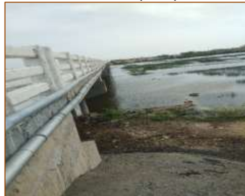
Side View of Major Bridge at km. 388+760 (LHS)
