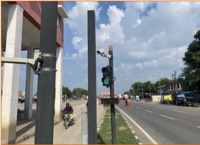
Toll Signal light
