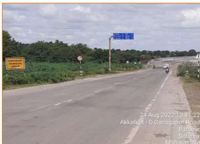
Start of the Project Highway at km. 99+400
