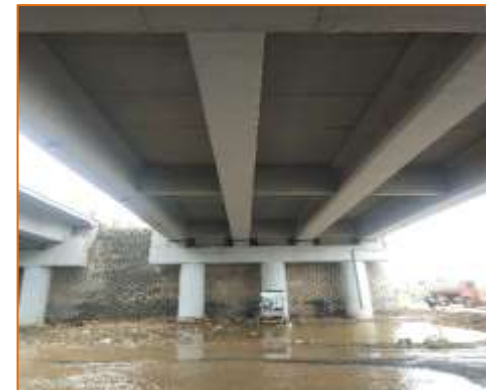
Bottom View of VUP at km. 12+420
