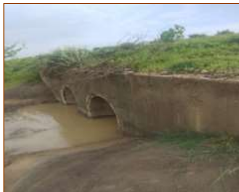
HPC at km. 487+054 (RHS)
