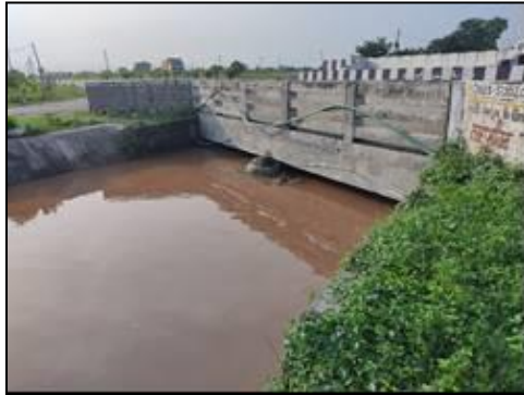
Minor Bridge at km. 35+812 (Existing Structure View)
