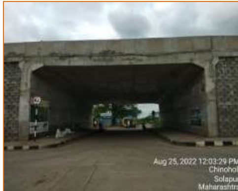
Side View of LVUP at km. 125.055 (RHS)
