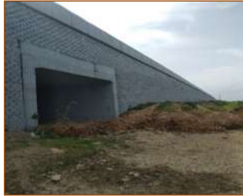
VUP at km. 393+695 (RHS)
