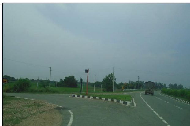
Major Junction at km. 1+250 (LHS)
