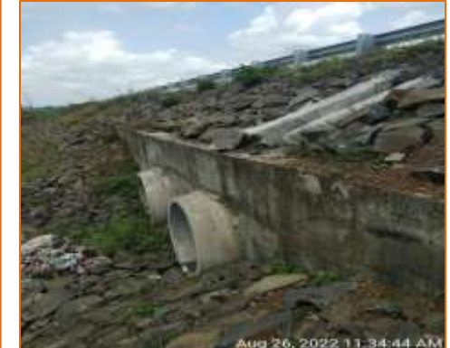
Pipe Culvert at km. 113.155-LHS (Widening)
