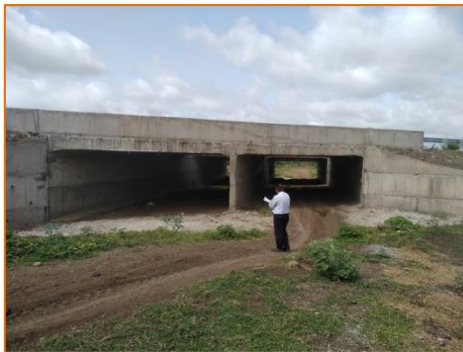
New Minor Bridge at km. 296.580
