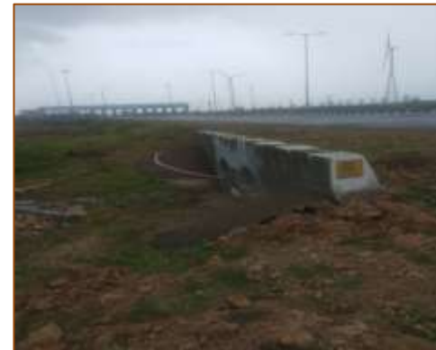
HPC at km. 409+195 (LHS)
