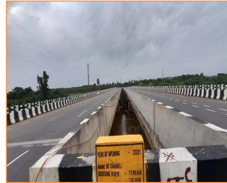
View of Major Bridge at km. 51+929
