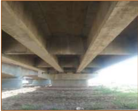
Bottom of MJB - New at km. 433+276 (LHS)
