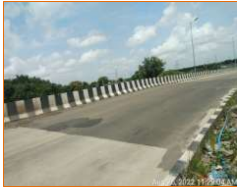
LVUP at km. 114.080 (LHS)
