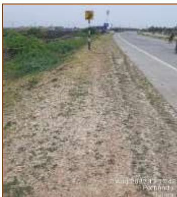
From km. 408+000 to km. 409+000 (RHS)
