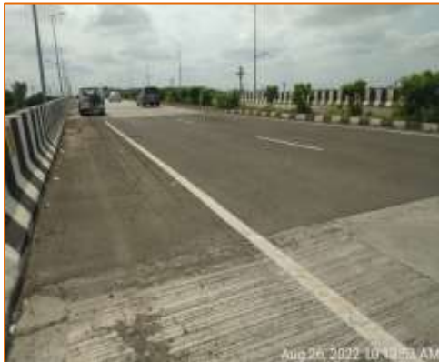
LVUP at km. 132.025 (RHS)
