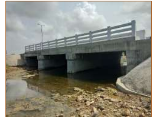
Side View of Minor Bridge at km. 480+171 (RHS) - New
