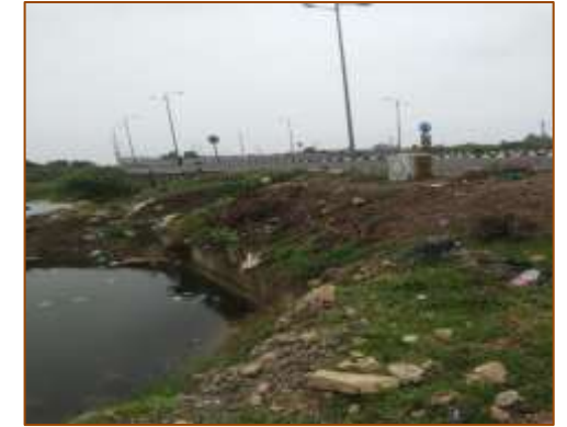
HPC at km. 391+096 (RHS)
