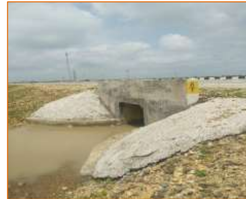
Box culvert at km. 7+240 (LHS)
