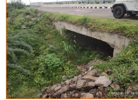
Box Culvert at km. 311.734
