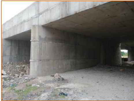
Widening of Existing Minor Bridge at km. 281.277
