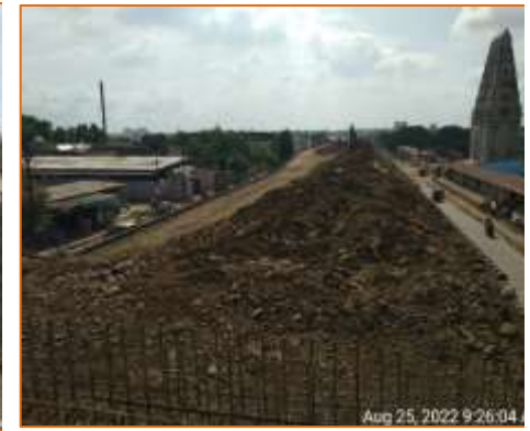
Filling work of Flyover is in progress at km.136.857 @ Akkalkot side (BHS)
