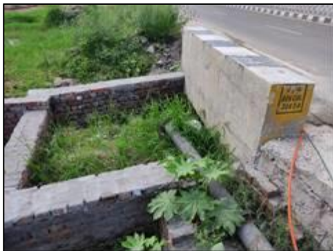
Box Culvert at km. 6+650
