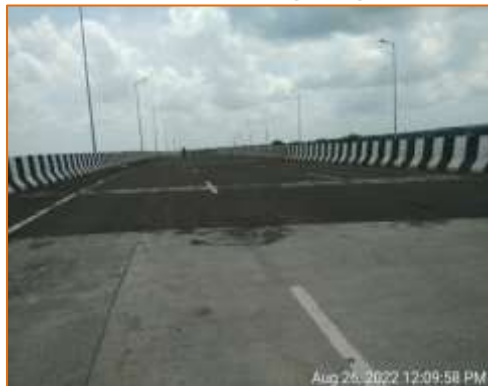
BC surface of Flyover at km. 102.700 (RHS)
