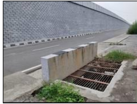
Box Culvert at km. 2+531
