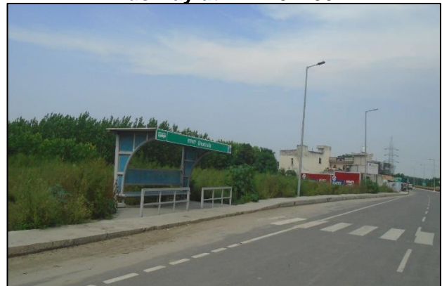
Bus Bay at km.69+200
