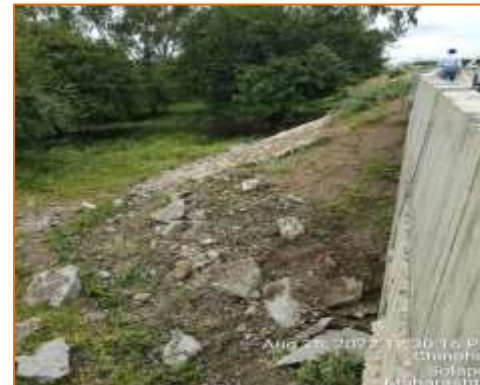
Rubble pitching pending @ A1 side of MNB at km. 124.337 (RHS)
