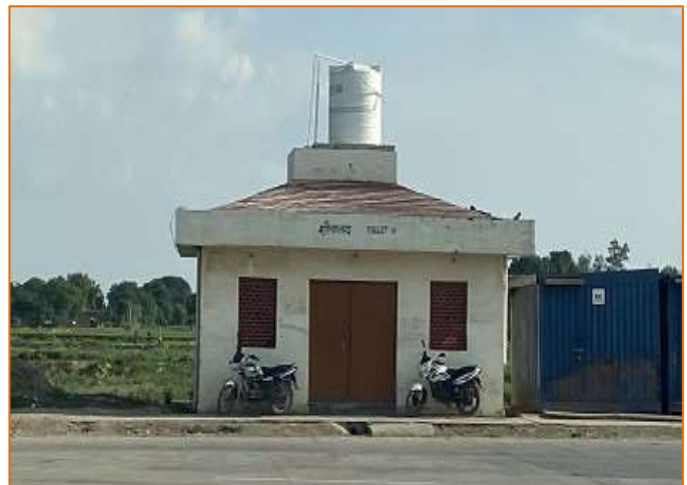
Toilet Block at Toll Plaza
