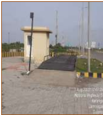
Static Weigh Bridge
