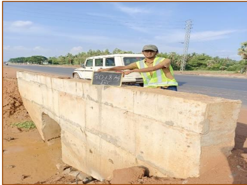
Box Culvert at km. 30+874
