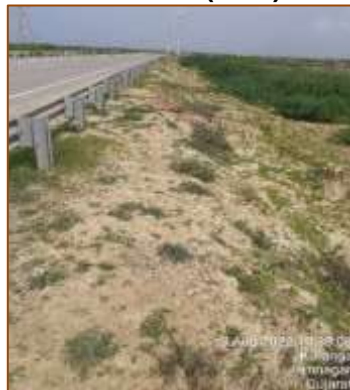
From km. 466+000 to km. 467+000 (RHS)
