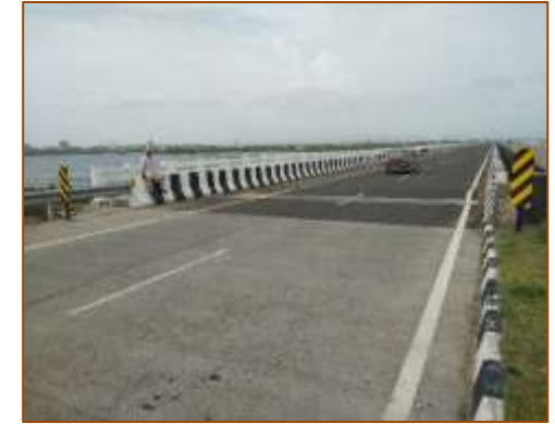
Wearing Coat of MJB at km. 386+750 (LHS)
