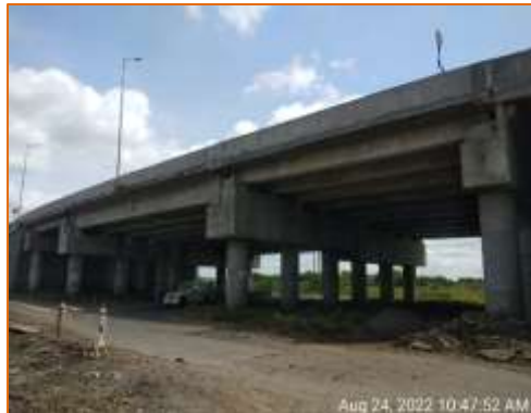
Side View of Flyover at km. 99.900 (LHS)
