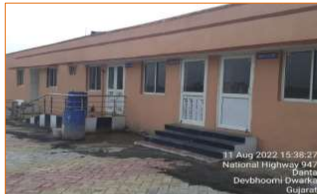
Highway / Medical / Traffic Post at Toll Plaza
