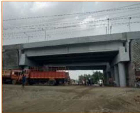
Side View of VUP at km. 55+300 (LHS)
