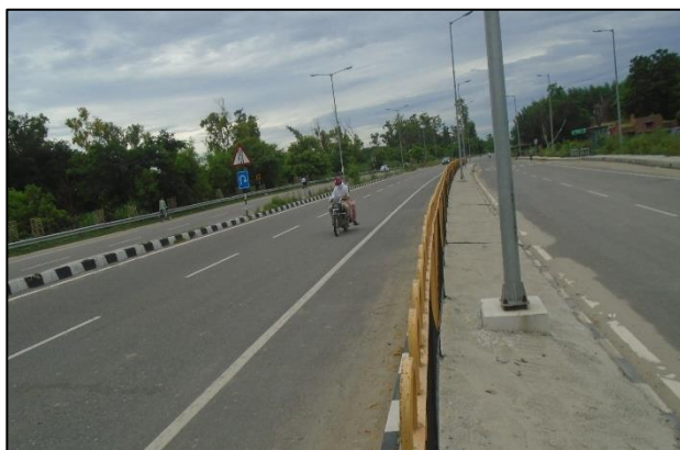
Pedestrian Guard Rail at km. 69+400
