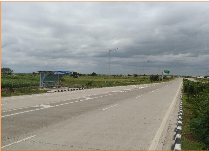
Bus Bay on service road at km. 305+800
