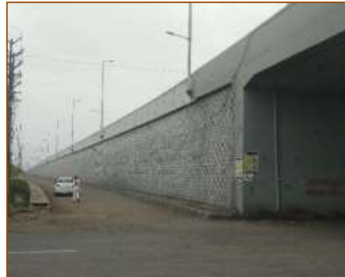
VUP at km. 400+681 (RHS) at A1 side
