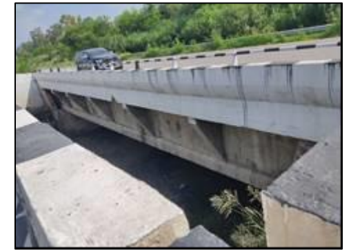
Minor Bridge at km. 63+615 (New Structure View)
