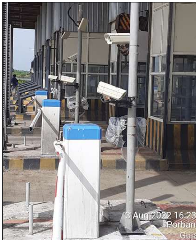
Figure 9-8 LPIC and AVC cameras
