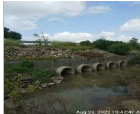
Pipe Culvert at km. 124.106 - RHS (Widening)
