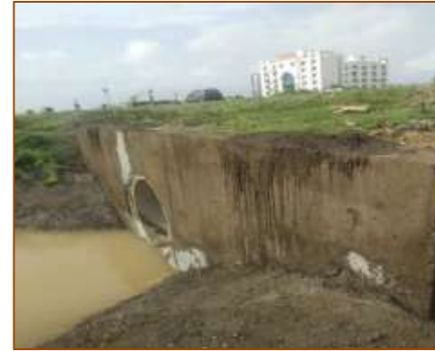
HPC at km. 490+350 (LHS)
