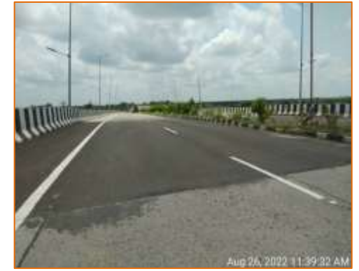
Good BC surface of LVUP at km. 111.260 (RHS)
