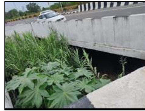
Minor Bridge at km. 78+636 (Structure View)
