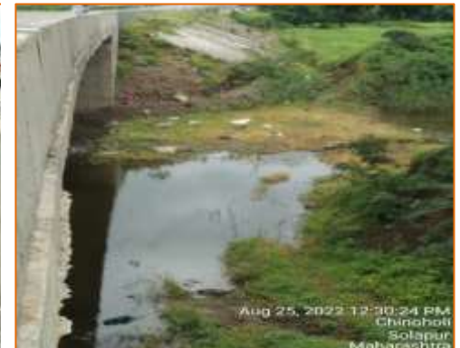
Rubble pitching pending @ A2 side of MNB at km. 124.337 (RHS)
