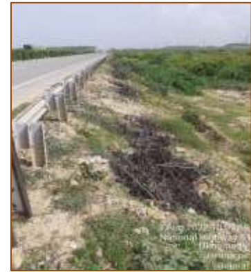
From km. 476+000 to km. 477+000 (RHS)
