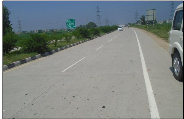
Rigid Pavement at km. 41+000
