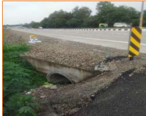
HPC at km. 66+010 (LHS)
