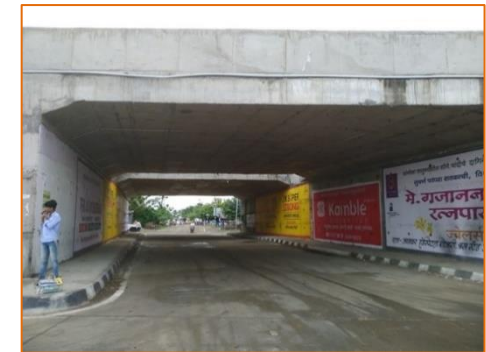
Light Vehicular Underpass at km. 298.613
