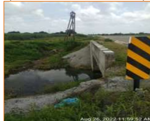
Box culvert at km. 105.290 - RHS (New Construction)
