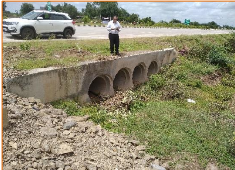
Pipe Culvert at km. 276+190
