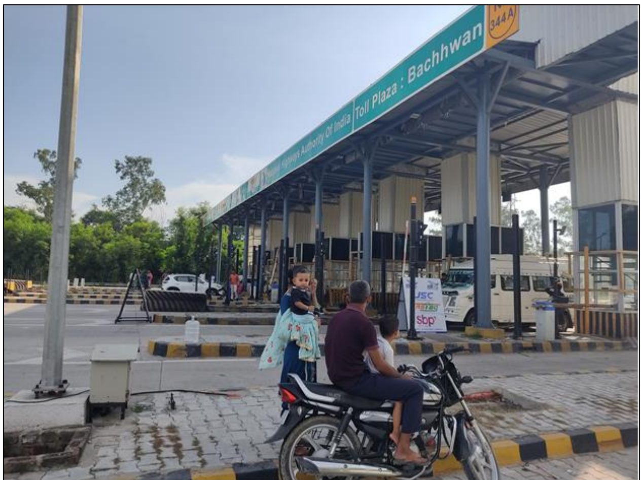
Figure 9-2 View of Bachhwan Toll Plaza (km. 70+240)
