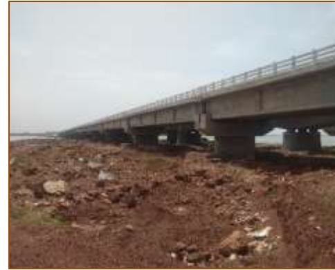
Major Bridge - km. 433+295 (RHS) side view
