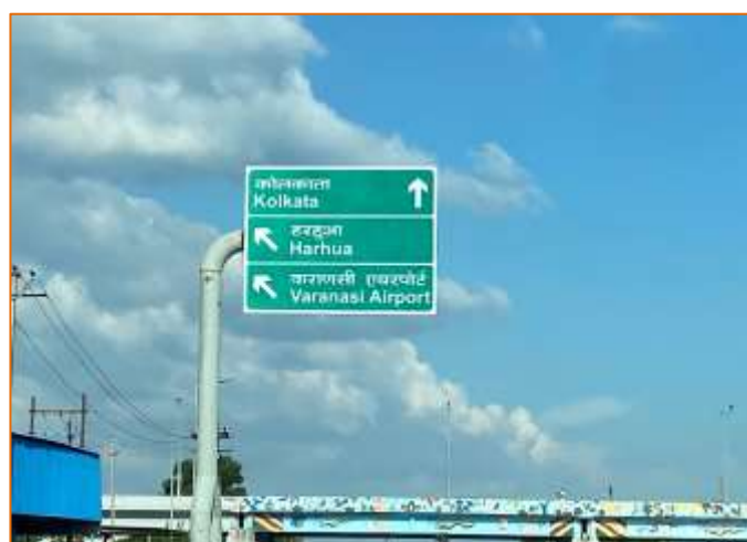
Cantilever Gantry Sign at km. 782+500
