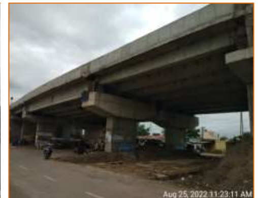
Side View of Flyover at km. 130.650 (RHS)
