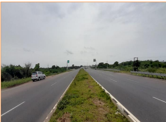
Pavement Condition at km. 55+100
