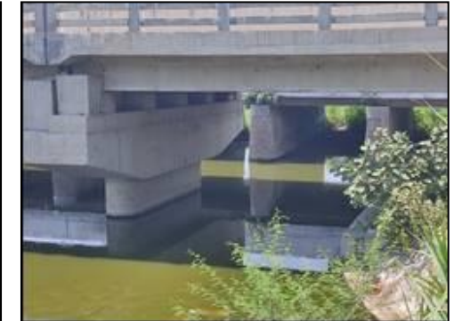
Major Bridge at km. 59+381 (Substructure and Super structure)
