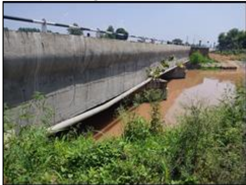
Minor Bridge at km. 48+323 (Existing Structure View)
