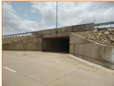
Pedestrian Underpass at km. 284.500
