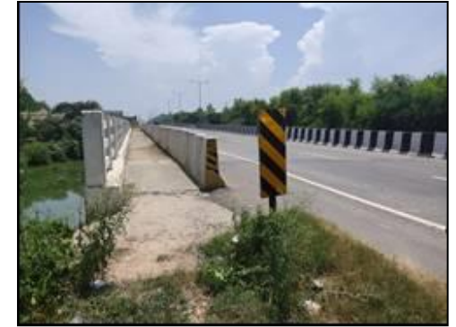
Minor Bridge at km 59+237 (top view)
