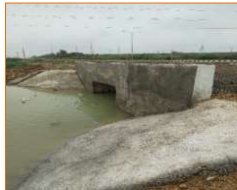
Box culvert at km. 11+950 (RHS)
