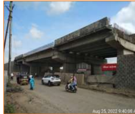
Side View of Flyover at km. 136.857 (LHS)
