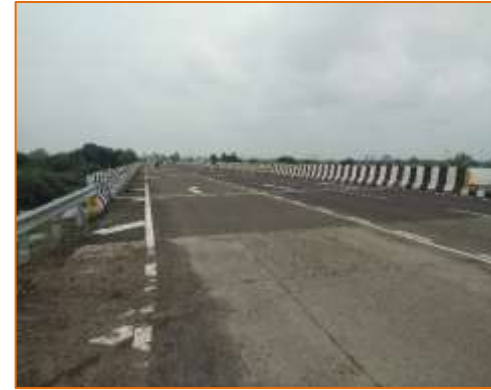
Wearing Coat of Major Bridge at km. 54+855 (RHS)
