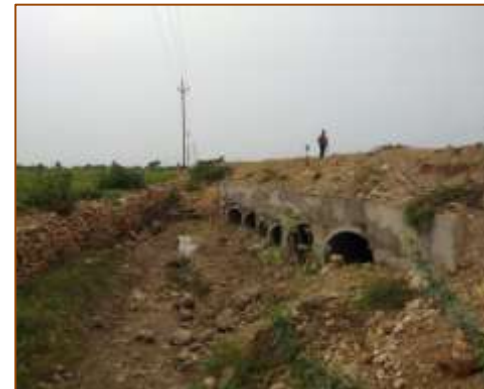
HPC at km. 456+200 (LHS)
