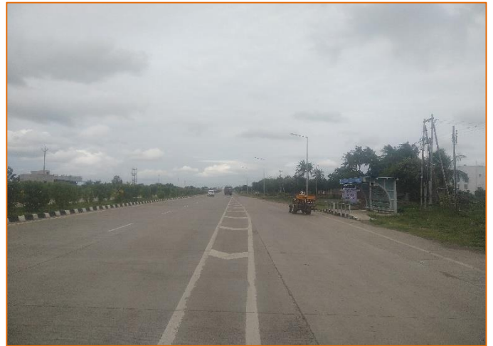
Bus Bay at km. 301+600 (Dighewadi)
