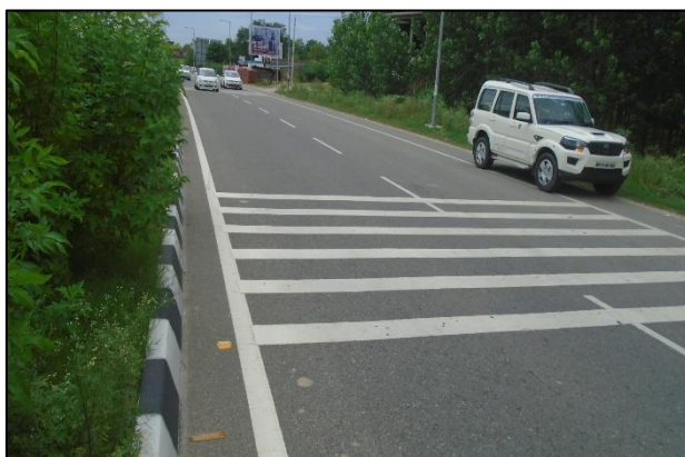
Road Marking at km. 70+000 (RHS)
