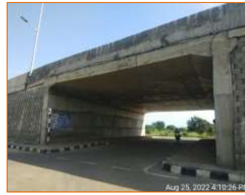
Side view of LVUP at km. 111.260 (RHS)
