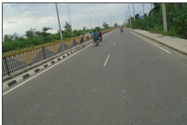
Pedestrian Guard Rail at km. 69+400
