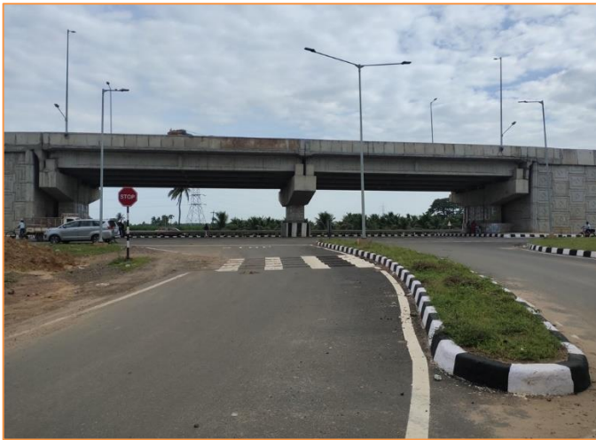
Highway Lighting at km. 45+645
