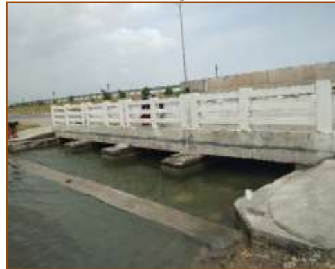
Side view of Minor Bridge at km. 406+170 (RHS) - Widening
