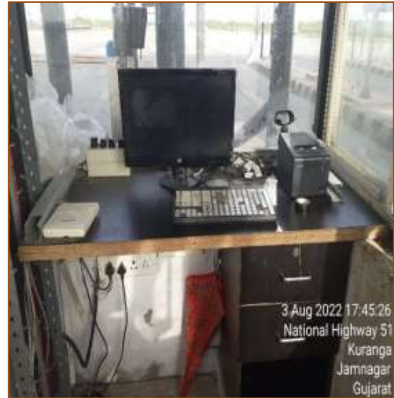
TP-2 at km. 470+875
