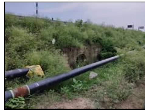
HP Culvert at km. 1+135
