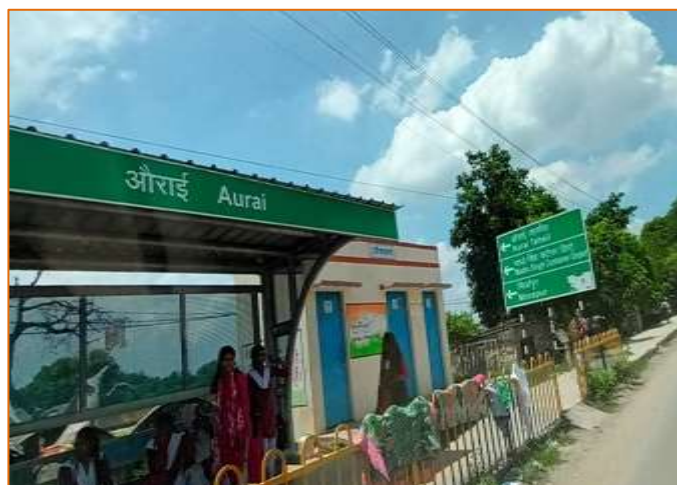
Toilet Block at km. 754+130
