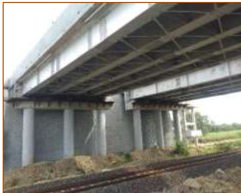
Side View of ROB at km. 393+642 (RHS)
