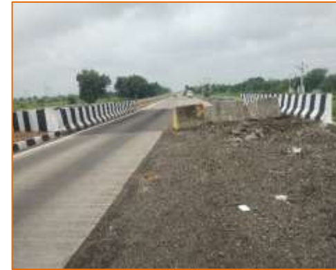
MCW pending (1-lane) of Minor Bridge (New) at km. 51+293 (LHS)
