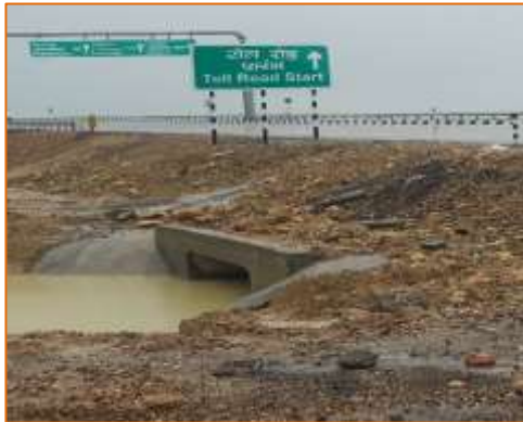
Box culvert at km. 0+060 (LHS)
