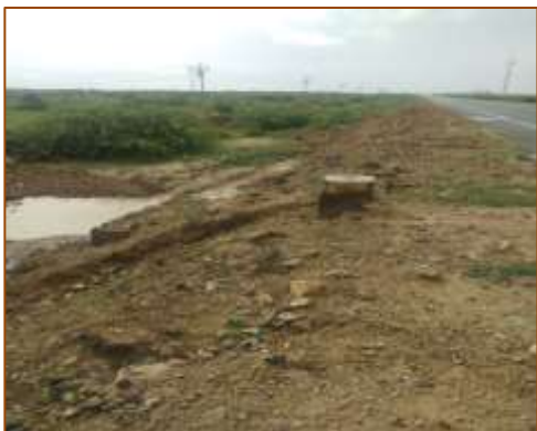
HPC at km. 487+054 (LHS)
