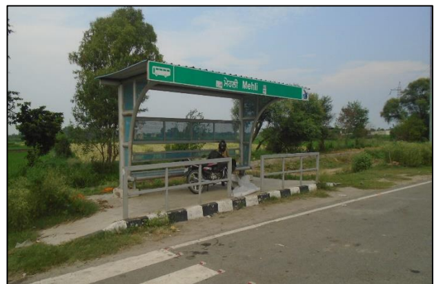
Bus Bay at km. 10+255
