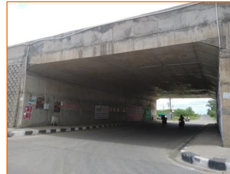
Light Vehicular Underpass at km. 285.432
