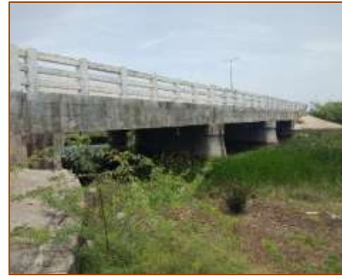
Side view of Minor Bridge at km. 434+974 (RHS) - Widening
