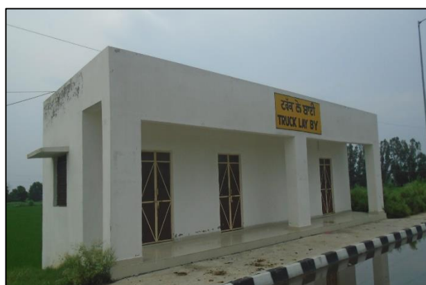
Truck Lay-Bye at km. 1+600
