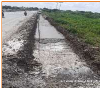
km. 133.300 WIP (RHS)
