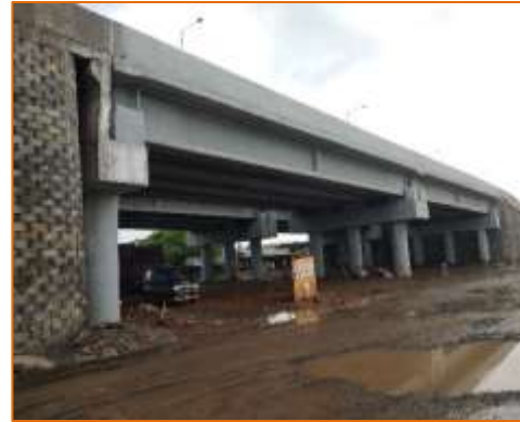
Side View of VUP (Limdi) at km. 23+120 (LHS)
