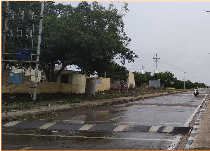
Built-up Drain at km. 314+735
