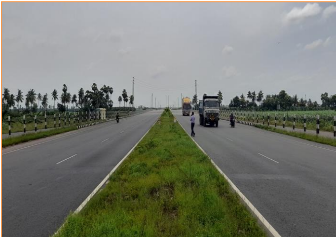
Pavement Condition at km. 41+200
