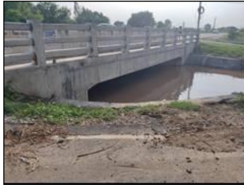
Minor Bridge at km. 35+812 (New Structure View)
