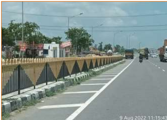
Pedestrian Guard Rail at km. 727+900
