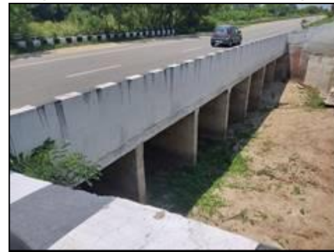
Minor Bridge at km. 57+981 (Existing Structure View)
