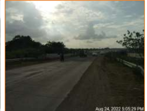
View of MNB at km. 99.586 (LHS)
