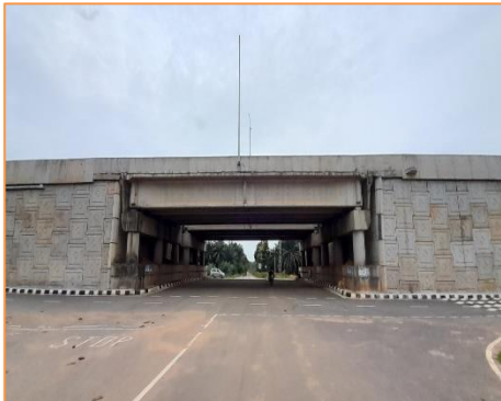
View of VUP at km 63+466
