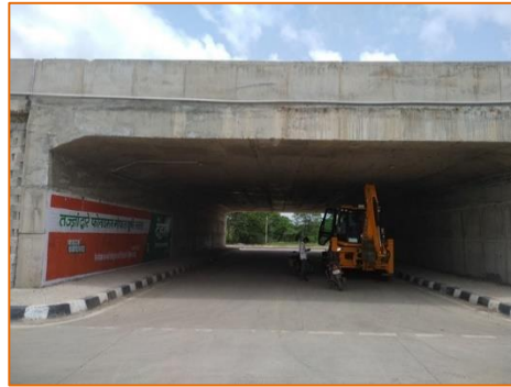
Light Vehicular Underpass at km. 288.116
