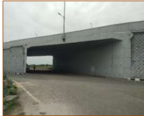
VUP at km. 397+096 (RHS)
