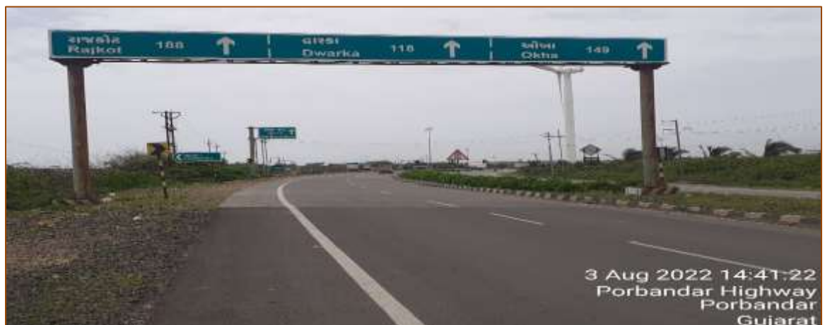
Figure 2-2 Start of project highway at km. 379+100
