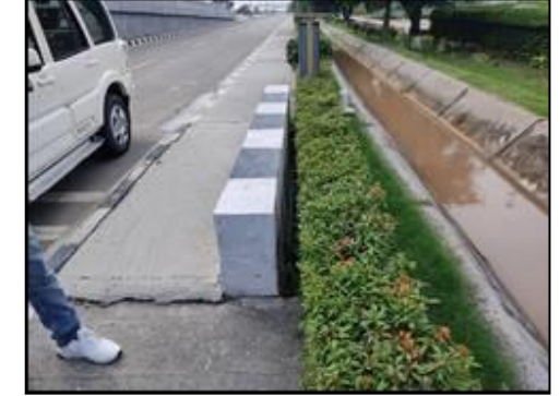
HP Culvert at km. 6+874
