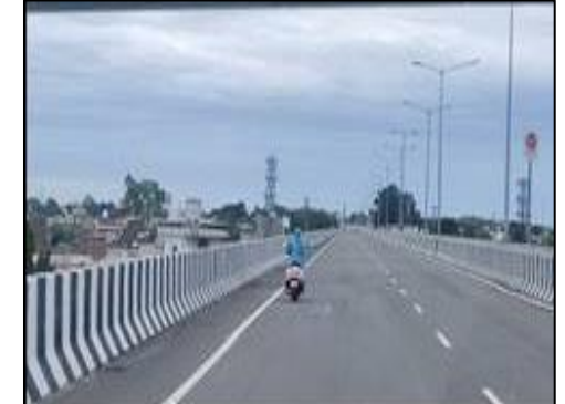
Elevated Structure at km. 25+319
