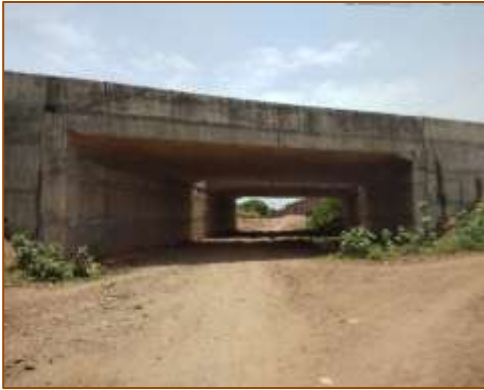
LVUP at km. 381+600 (RHS) - Under COS
