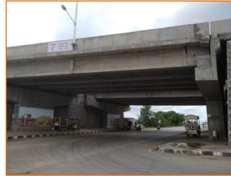
Vehicular Underpass at km. 294.456
