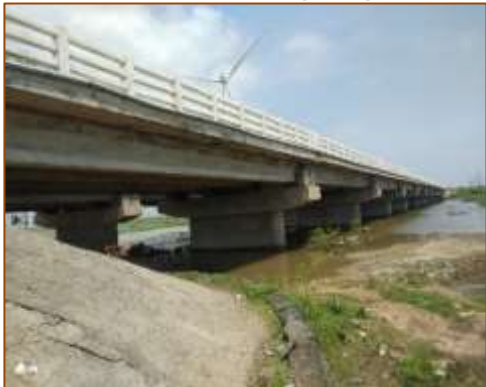
Side View of Major Bridge at km. 415+929 (LHS)
