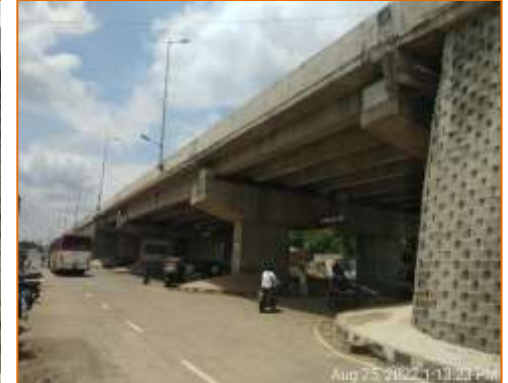
Side View of Flyover at km. 117.935 (RHS)
