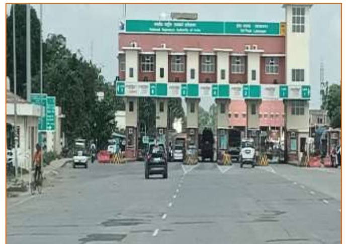
Toll Plaza including Admin Building at km. 747+822
