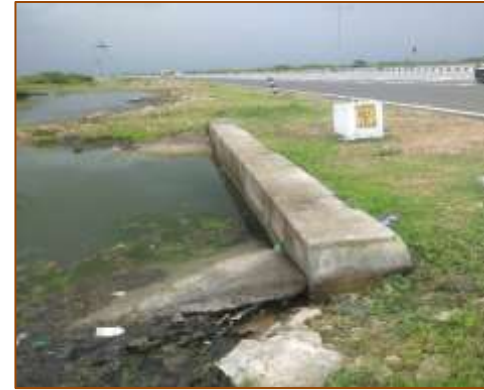
HPC at km. 391+096 (LHS)
