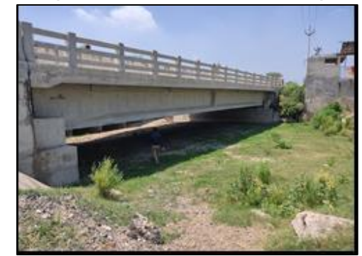
Minor Bridge at km. 57+981 (New Structure View)
