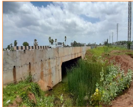
View of Minor Bridge at km. 26+850
