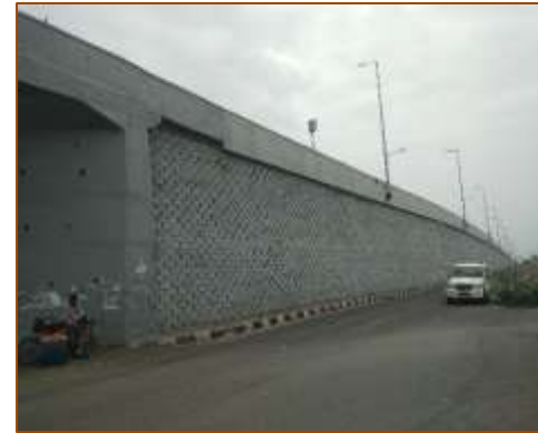
VUP at km. 397+096 (LHS) - Skew - A1 side
