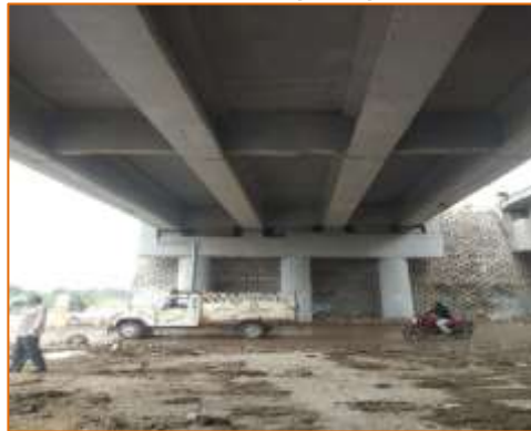
Bottom View of VUP at km. 55+300
