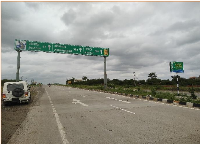
Cantilever Gantry Sign at km. 321+600
