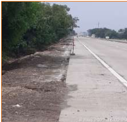
km. 32+450 Work in Progress
