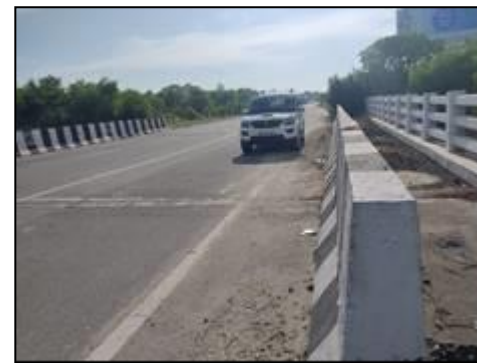
Minor Bridge at km. 71+727 (Top View)
