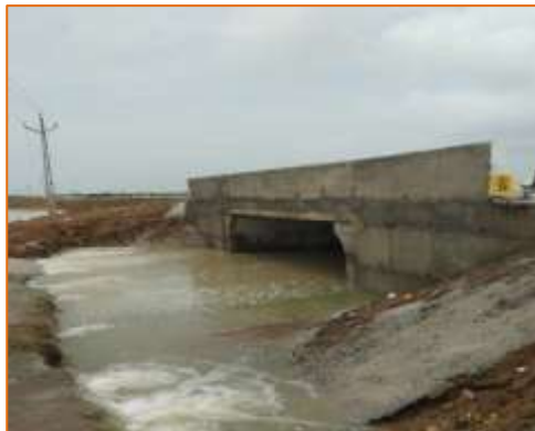
Side View of Minor Bridge at km. 9+880 (RHS)
