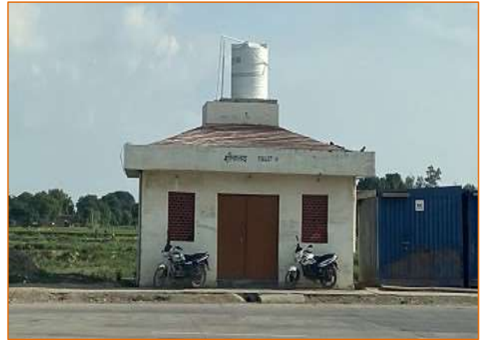
Toilet Block at Toll Plaza
