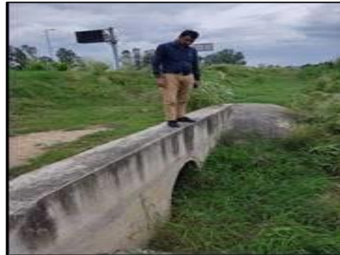
HP Culvert at km. 69+420
