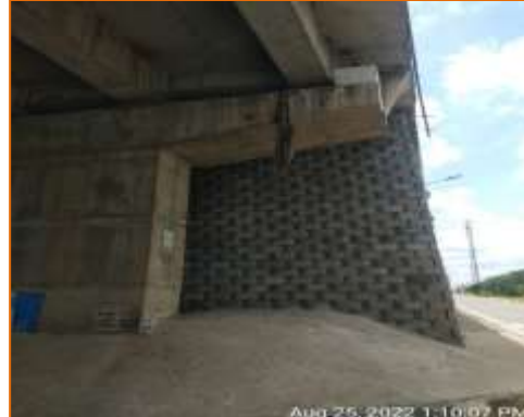
Hanging hessian cloth @ A2 cap of Flyover at km. 117.935 (RHS)
