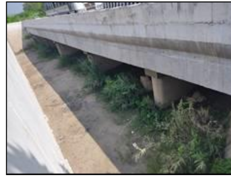
Minor Bridge at km. 64+791 (Existing Structure View)
