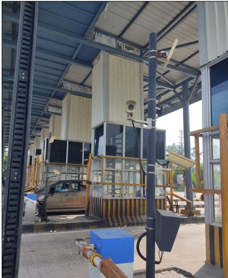
Figure 9-9 LPIC and AVC Cameras
