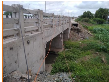
Reconstruction of Minor Bridge at km. 284.835
