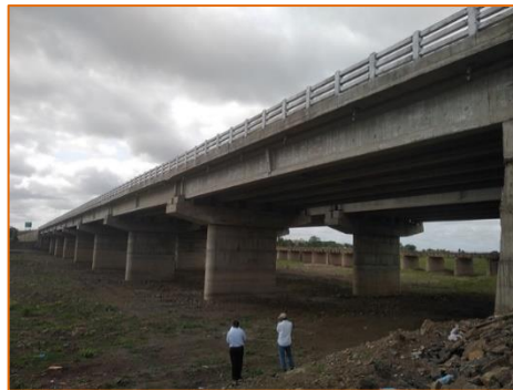
New Major Bridge at km. 298.190
