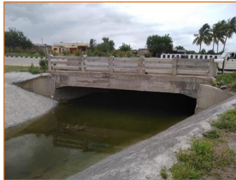
New Minor Bridge at km. 319.849 on LHS
