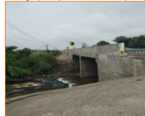
Side View of Minor Bridge at km. 54+945 (RHS)
