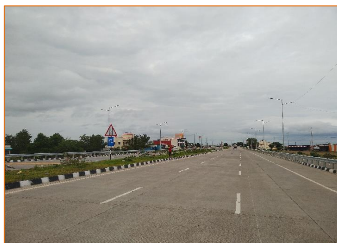
Road Markings at km. 286+600
