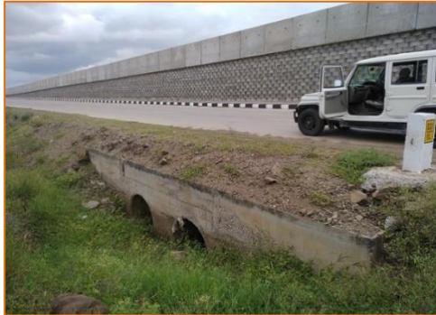
Pipe Culvert at km. 321.024
