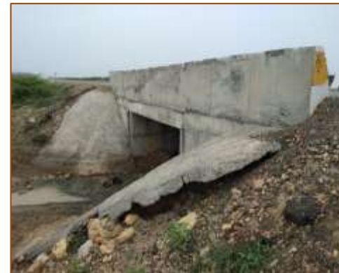
Slab culvert at km. 475+860 (LHS)
