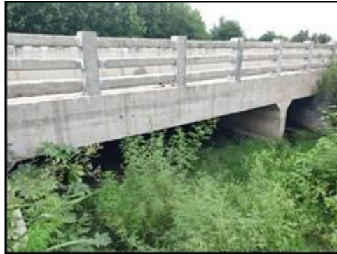
Minor Bridge at km. 74+361 (Structure View)
