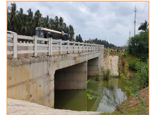
View of Minor Bridge at km. 30+774
