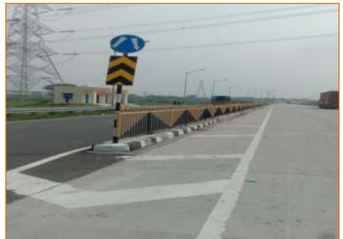
Pedestrian Guard Rail at km.766+600
