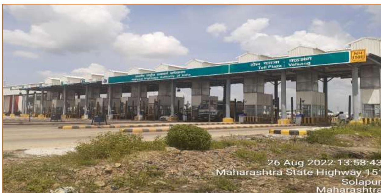
Figure 9-1 View of Valsang Toll Plaza
