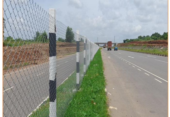
Chain fencing at km. 78+800
