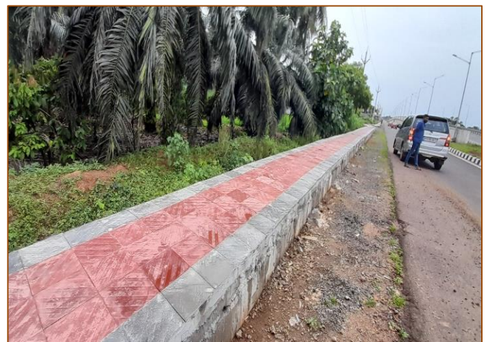
Built-up Drain cum footpath at km. 36+450
