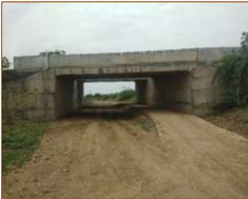
LVUP at km. 422+750 (RHS) - Under COS
