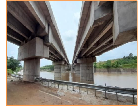
View of Major Bridge at km. 68+742
