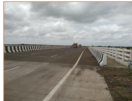
New Major Bridge at km. 280.420
