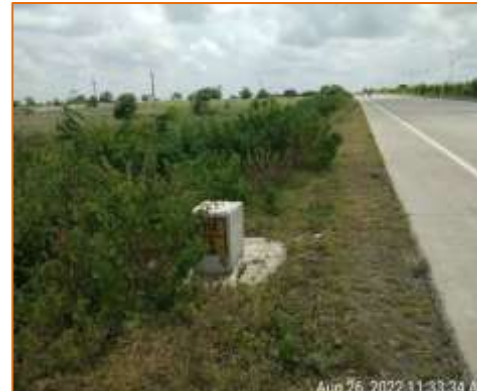
Pipe Culvert at km. 113.155 - RHS (Widening)
