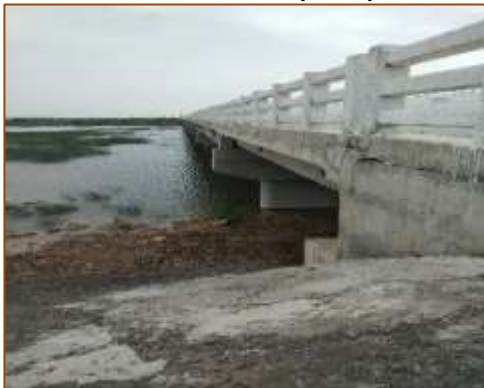
Side View of Major Bridge at km. 388+760 (RHS)
