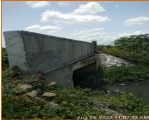
Box culvert at km. 101.823 - LHS (New Construction)
