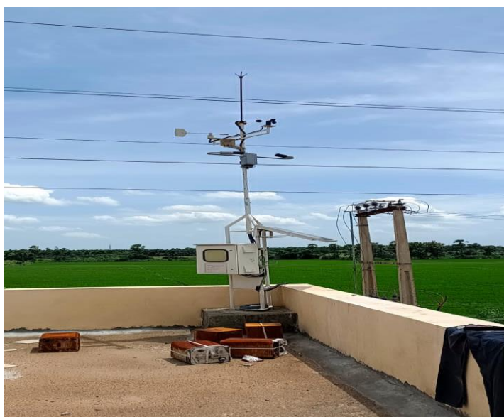
Figure 9-15 MET Equipment
