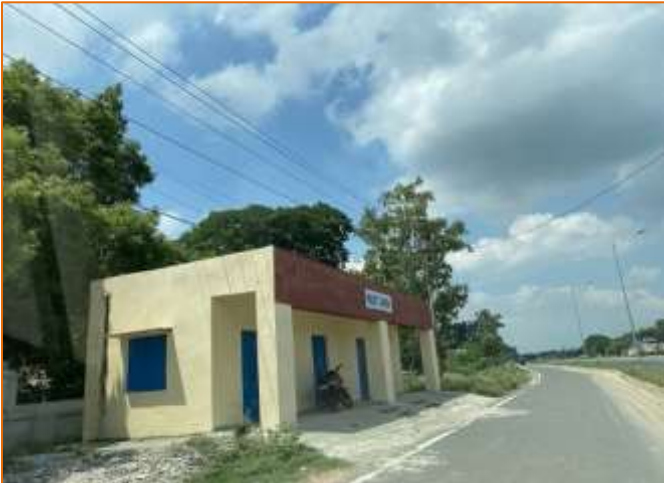
Rest Area at km. 727+800
