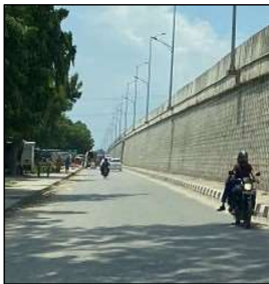
Service Road at km. 765+150
