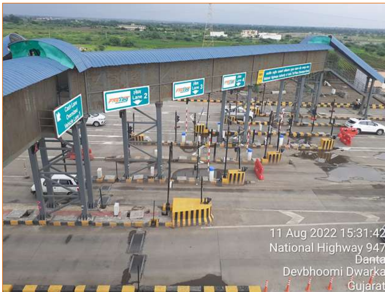
Figure 8-1 Views of Dharampur Dante Toll Plaza
