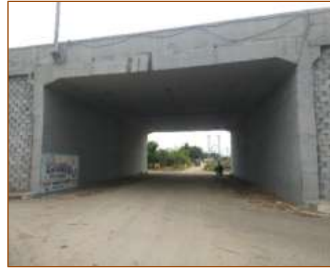
LVUP at km. 422+750 (LHS) - Under COS
