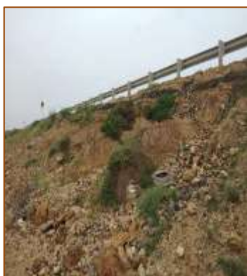
MJB at km. 474+405 (RHS)
