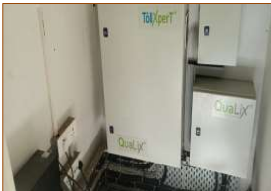
TP-1 at km. 409+500
