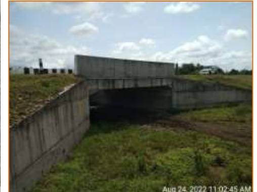
Side View of Minor Bridge at km. 101.260 (LHS)
