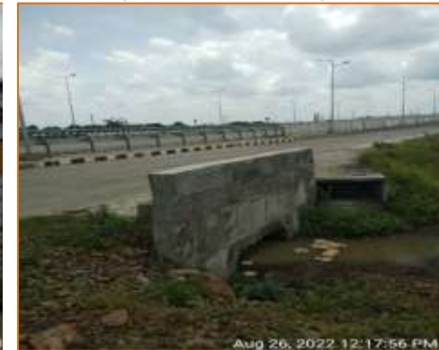
Box culvert at km. 133.524 - LHS (Reconstruction)
