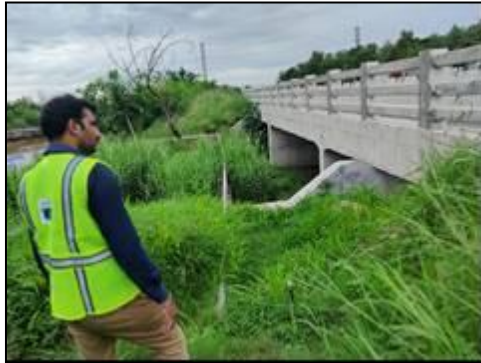
Minor Bridge at km. 74+173 (Structure View)
