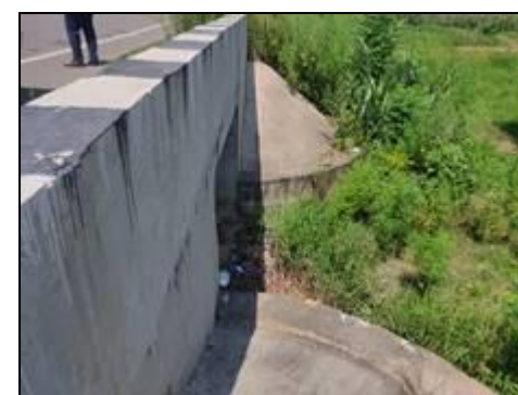
Box Culvert at km. 48+800
