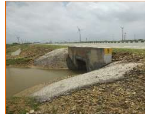
Box culvert at km. 7+240 (RHS)
