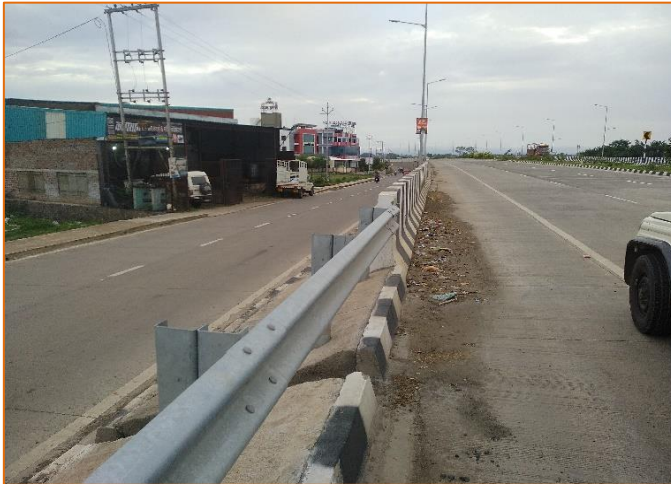
Crash Barrier at km. 285+650
