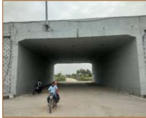
LVUP at km. 381+600 (LHS) - Under COS
