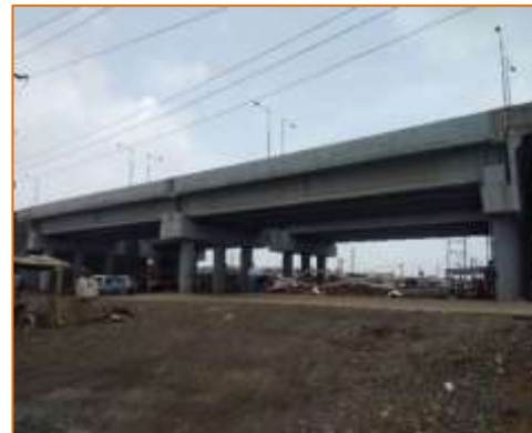
Side View of VUP at km. 12+420 (LHS)
