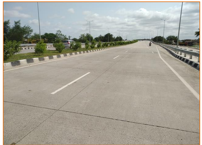
Start of Project Road at km. 276.000
