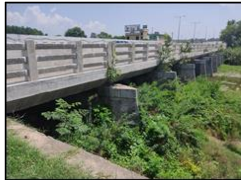
Major Bridge at km. 59+381 (Existing Structure View)
