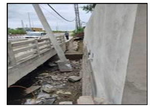
Minor Bridge at km. 80+045 (Structure View)
