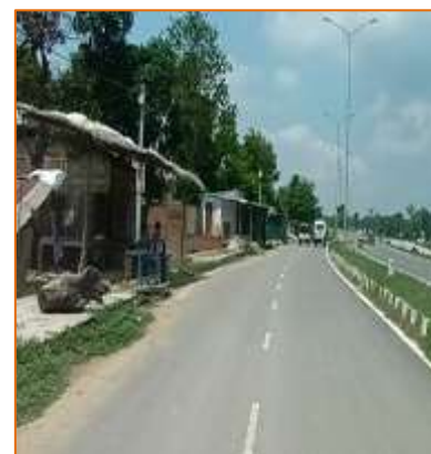
Service Road at km. 780+750
