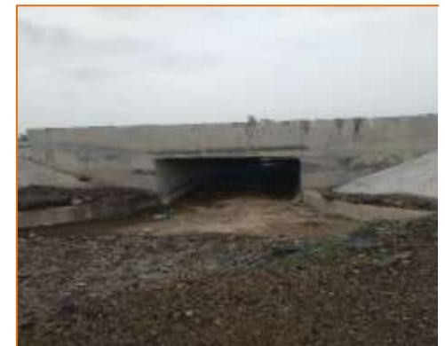
Box culvert at km. 62+720 (RHS)
