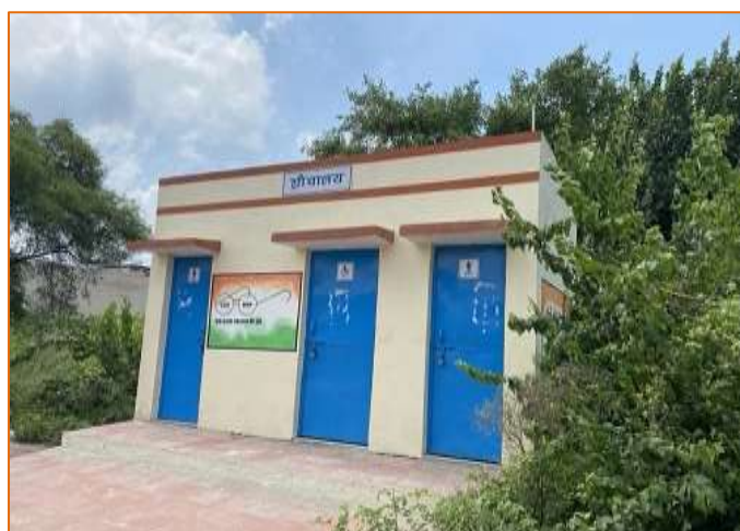
Toilet Block at km. 764+770
