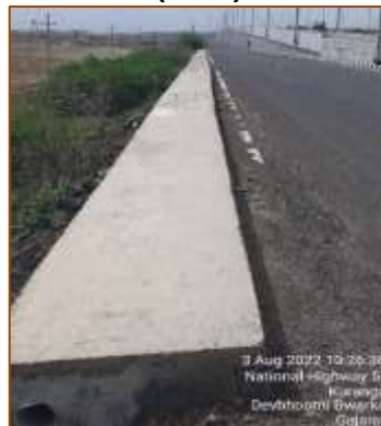
Built-up drain from km. 467+601 to km. 468+347 (RHS)
