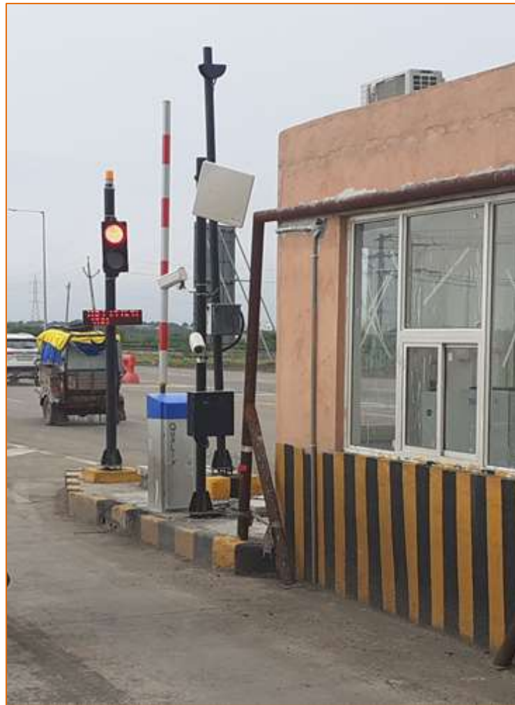
Figure 8-2 RFID Scanner located on pole
