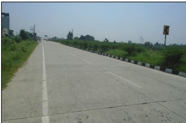
Rigid Pavement at km. 38+000
