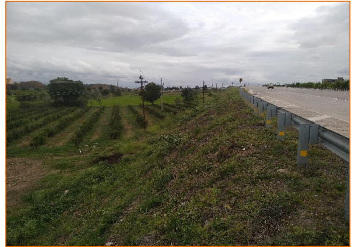
Crash Barrier at High Embankment Location
