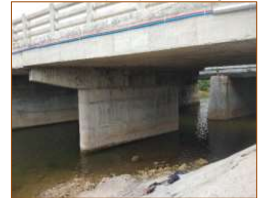
Bottom of Minor Bridge at km. 455+195 (RHS)
