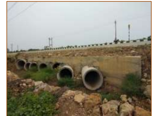
HPC at km. 456+200 (RHS)
