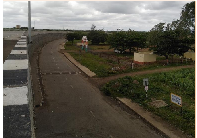
Built-up Drain at km. 299+350
