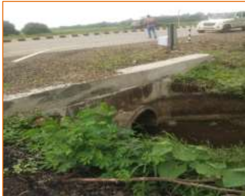
HPC at km. 66+010 (RHS)
