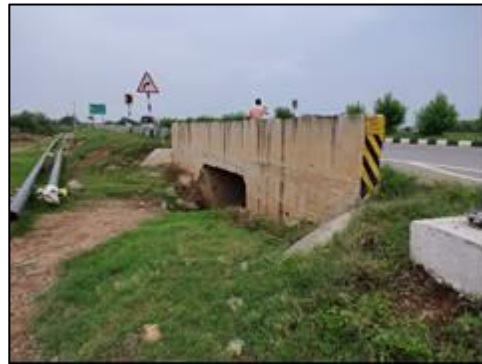
Box Culvert at km. 0+960
