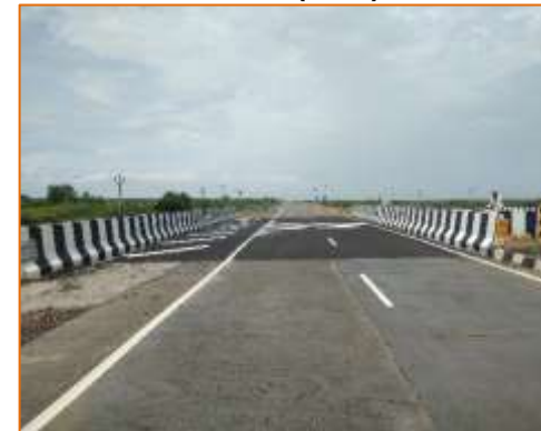
Wearing Coat of Minor Bridge at km. 3+010 (LHS)
