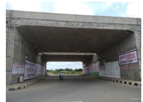
Vehicular Underpass at km. 287.300
