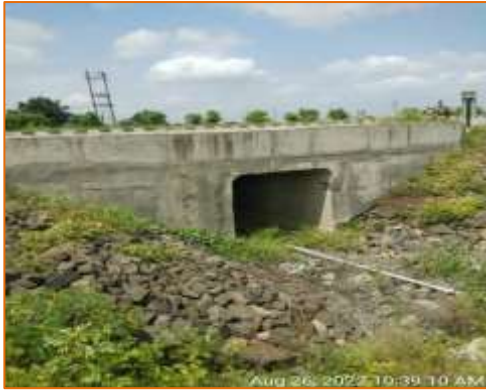
Box culvert at km. 125.495 - RHS (Reconstruction)
