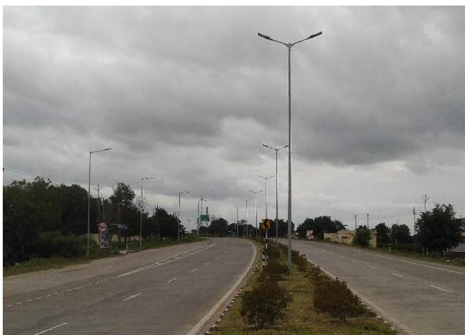
Highway Lighting at km. 313+700
