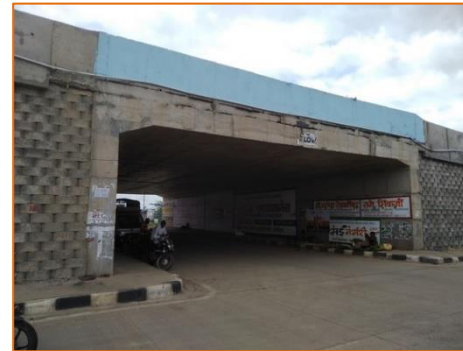
Light Vehicular Underpass at km. 283.165
