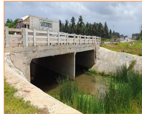
View of Minor Bridge at km. 28+782
