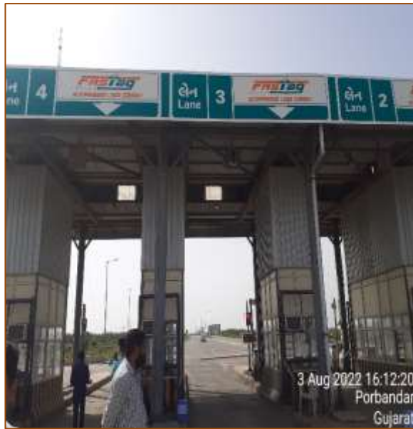
TP-1 at km. 409+500
