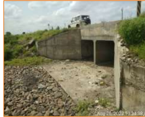
Box culvert at km. 126.643 - RHS (Reconstruction)
