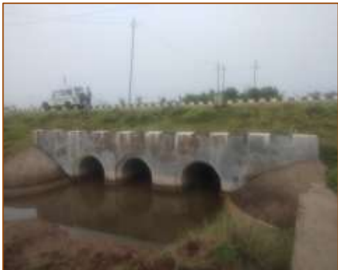
HPC at km. 437+025 (LHS)
