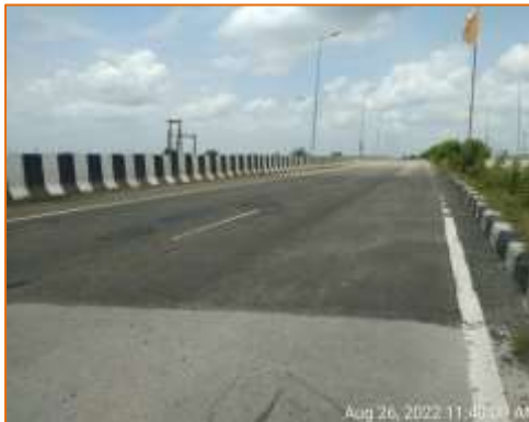
LVUP at km. 111.260 (LHS)
