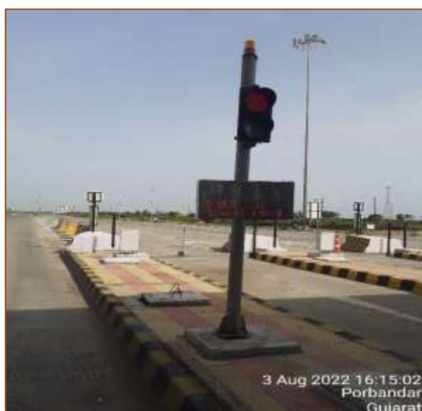
TP-1 at km. 409+500
