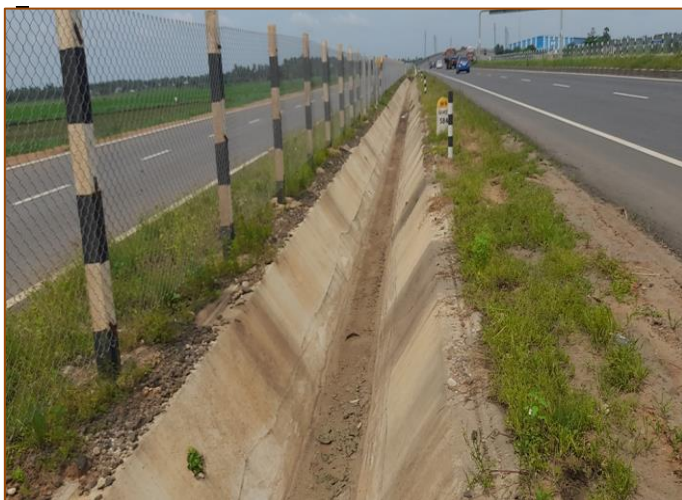
V Drain at km. 78+900
