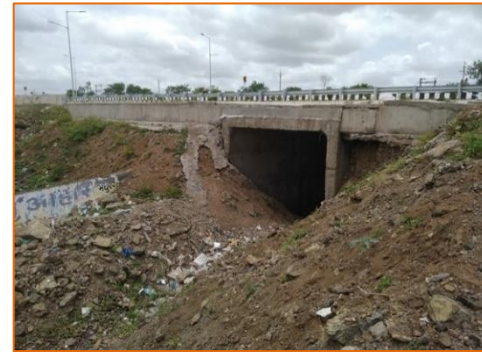
Box Culvert at km. 284+112
