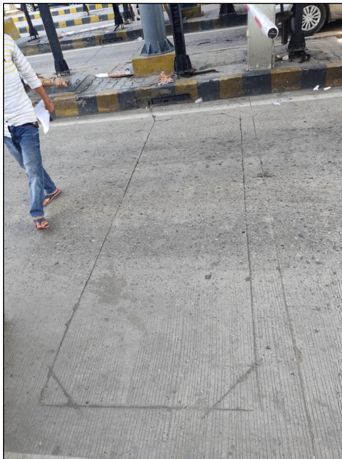
Figure 9-6 Inductive loop
