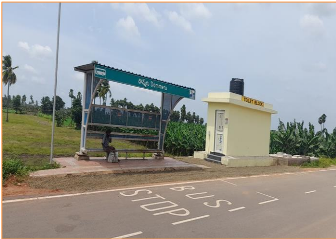
Bus Bay with Shelter at km. 79+200
