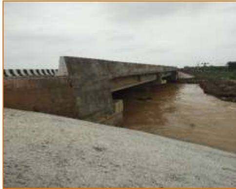
Side view of Minor Bridge at km. 22+495 (LHS)
