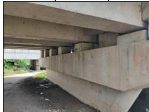
Minor Bridge at km. 71+174 (Substructure and Super structure)
