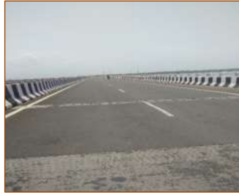
Major Bridge - km. 433+295 (LHS) Wearing Coat
