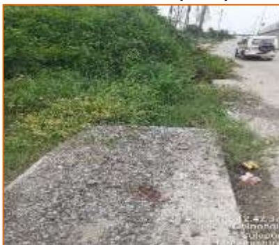
km. 121.470 (RHS) partially completed
