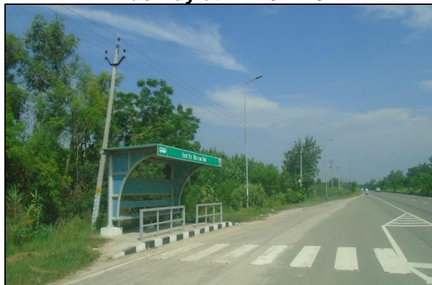
Bus Bay at km. 62+900
