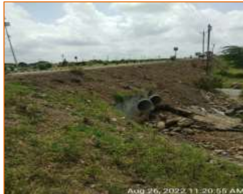
Pipe Culvert at km. 117.423 - LHS (Widening)
