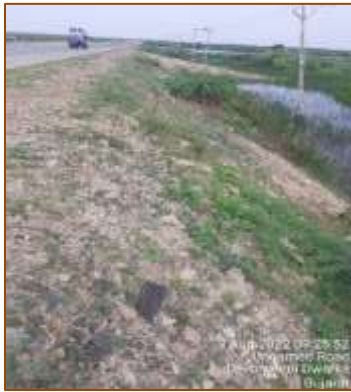
From km. 492+000 to km. 493+000 (RHS)
