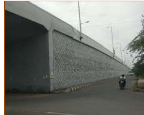
VUP at km. 400+681 (LHS) at A1 side
