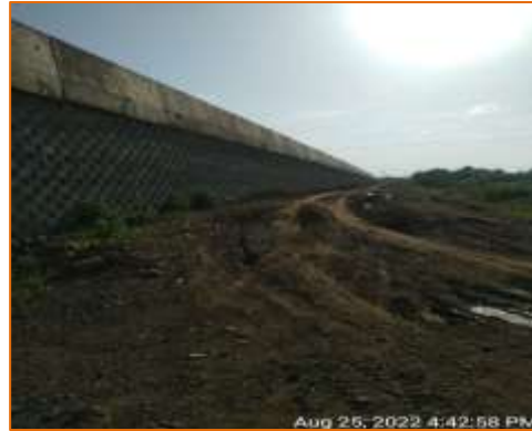
RE Block Wall @ A2 side of PUP at km. 104.820 (RHS)
