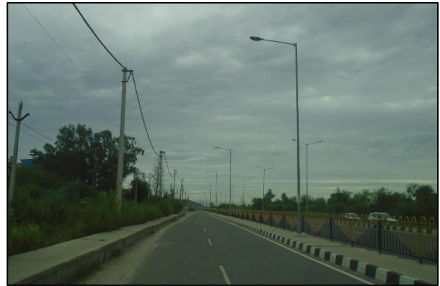
Street Lighting at Service Road
