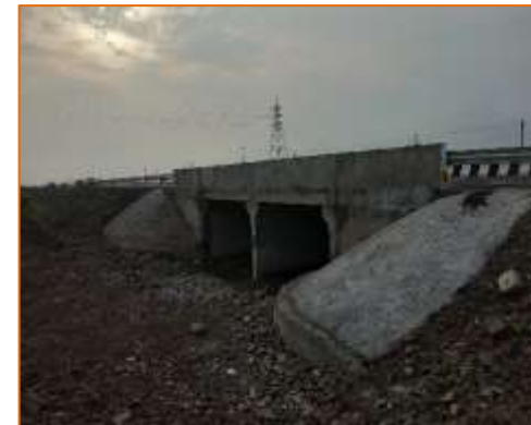
Side View of Minor Bridge at km. 47+700 (RHS)
