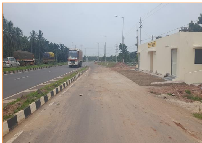
Truck Lay bye at km. 41+500
