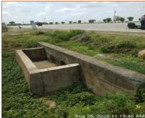
Pipe Culvert at km. 117.423 - RHS (Widening)
