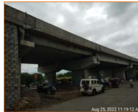
Side View of Flyover at km. 130.650 (LHS)
