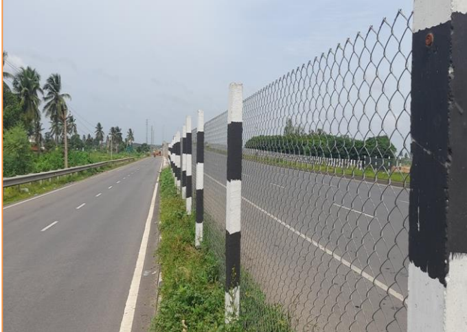
Chain fencing at km. 85+150
