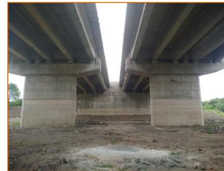
New Major Bridge at km. 298.190
