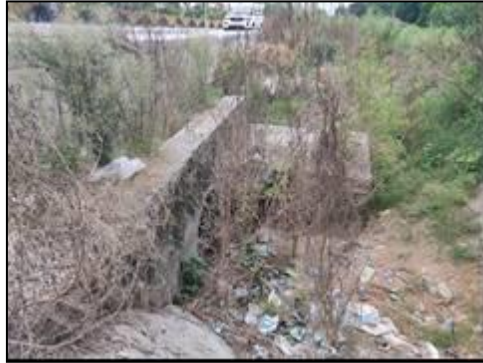
HP Culvert at km. 80+569
