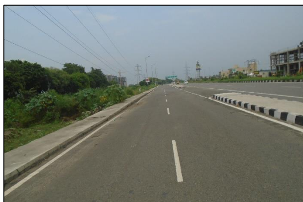
Service Road at km. 0+630 (LHS)
