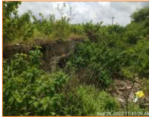
Pipe Culvert at km. 109.578 - LHS (Widening)
