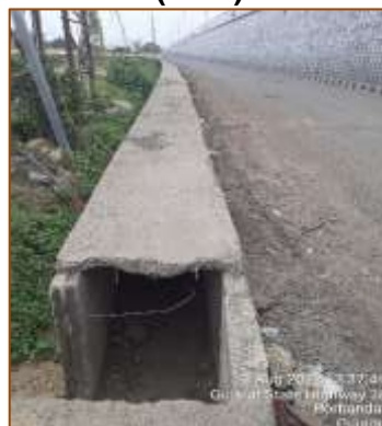
Built-up drain from km. 400+319 to 400+700 (LHS)
