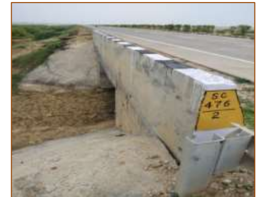
Slab culvert at km. 475+860 (RHS)
