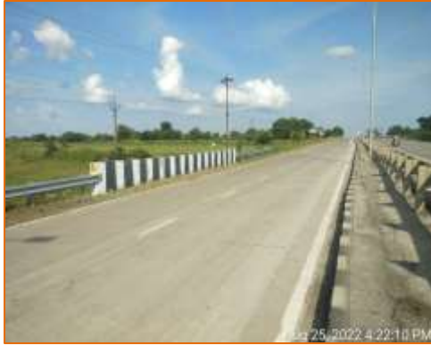
Good PQC surface of SR at MNB at km. 110.930 (RHS)
