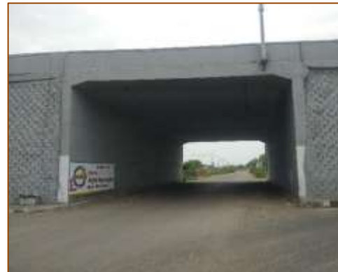
VUP at km. 396+865 (RHS)
