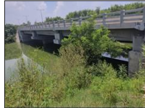
Major Bridge at km. 59+381 (New Structure View)
