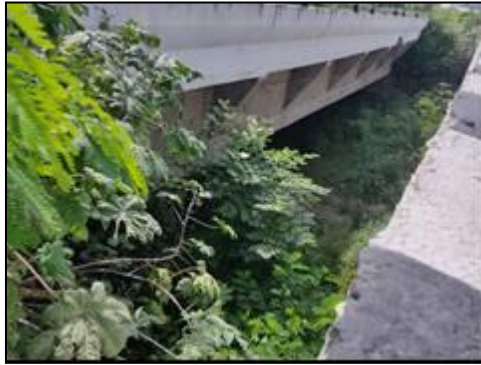
Minor Bridge at km. 66+020 (New Structure View)
