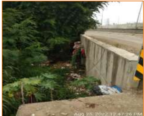
Side View of Minor Bridge at km. 121.678 (LHS)
