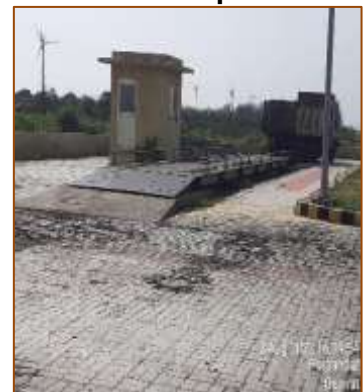
Static Weigh Bridge
