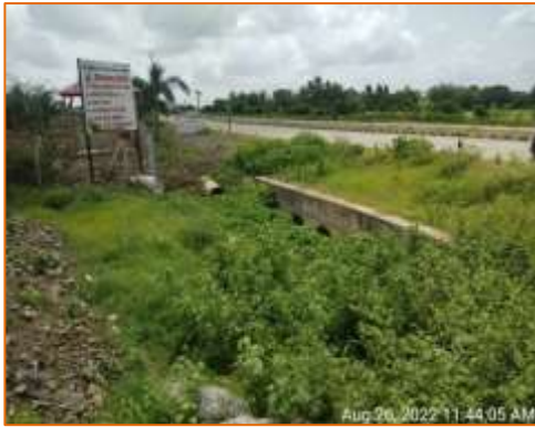
Pipe Culvert at km. 109.578 - RHS (Widening)
