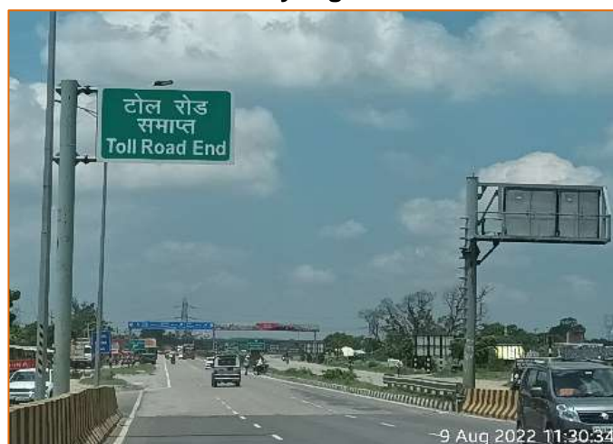
Cantilever Gantry Sign at km. 713+000.
