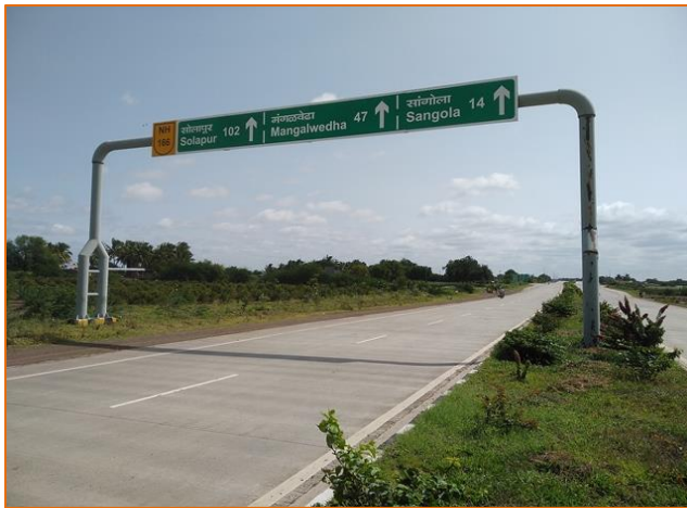
Start of Project Road at km. 276.000
