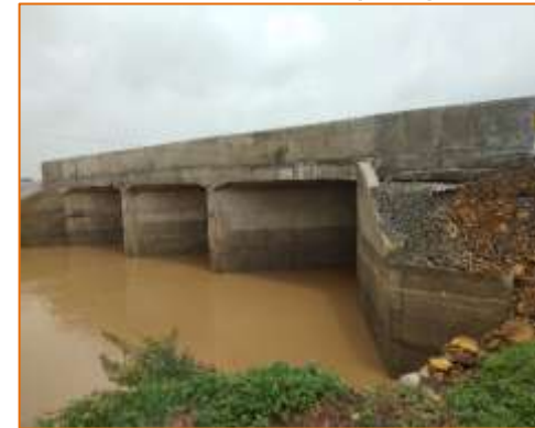
Side View of Minor Bridge at km. 21+955 (LHS)
