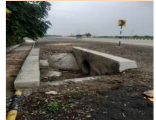
HPC at km. 70+640 (LHS)
