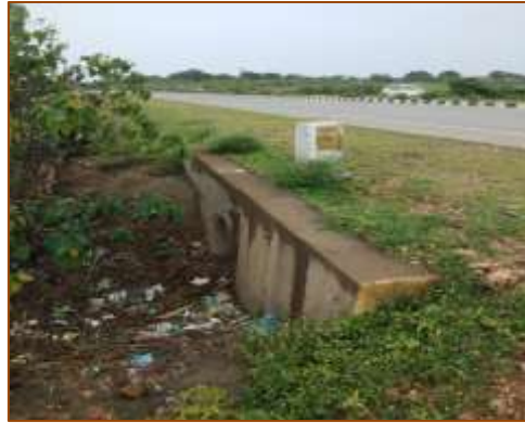
HPC at km. 380+328 (RHS)
