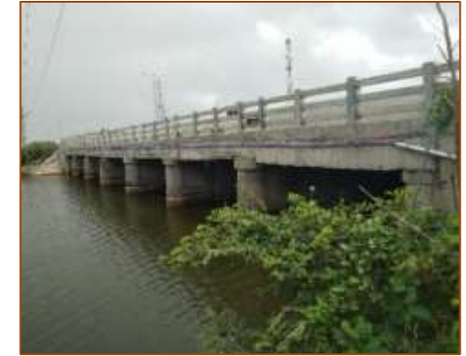
Side View of Minor Bridge at km. 450+241 (RHS) - Widening
