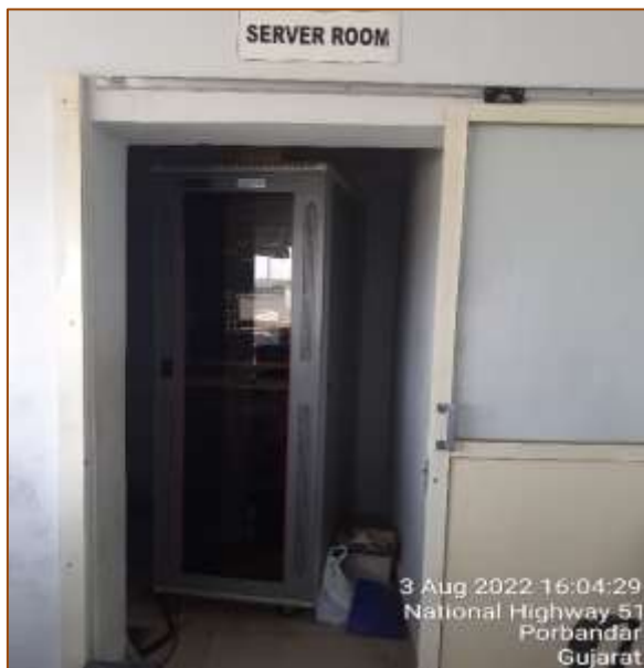
TP-1 at km. 409+500
