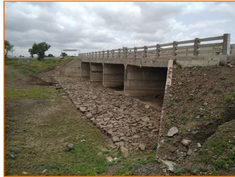
New Minor Bridge at km. 282.548
