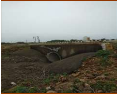
HPC at km. 380+328 (LHS)
