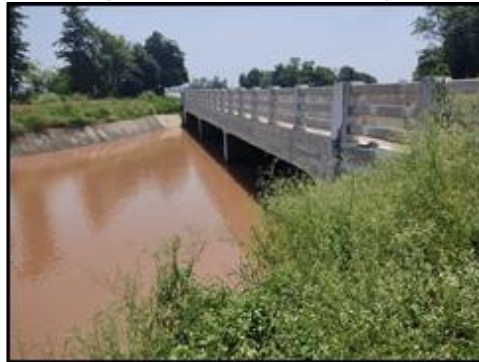
Minor Bridge at km. 48+323 (New Structure View)
