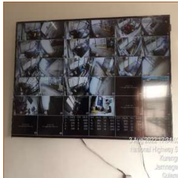
TP-2 at km. 470+875
