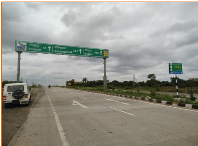
End of Project Road at km. 321.600
