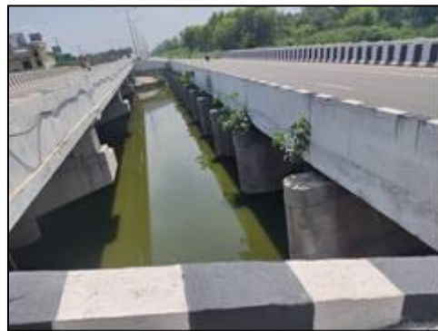
Major Bridge at km. 59+381 (Top View)
