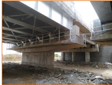
Rail Over Bridge at km. 294.125
