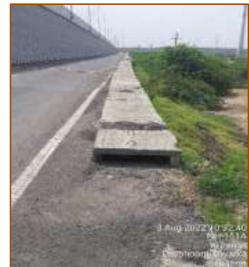
Built-up drain from km. 467+601 to km. 468+347 (LHS)
