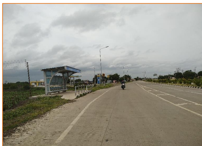
Bus Bay at km. 312+150 (Andhalgaon)
