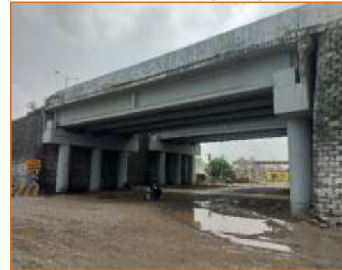
Side View of VUP at km. 57+975 (LHS)
