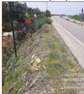
From km. 443+000 to km. 444+000 (RHS)
