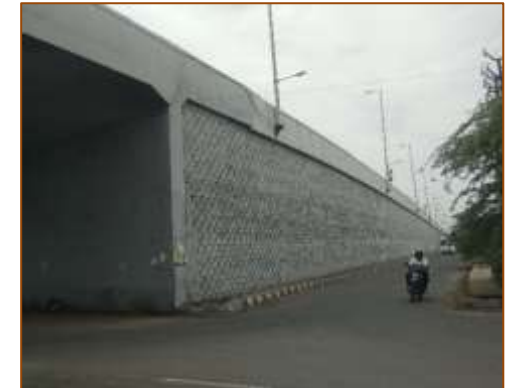
VUP at km. 400+681 (LHS) at A1 side
