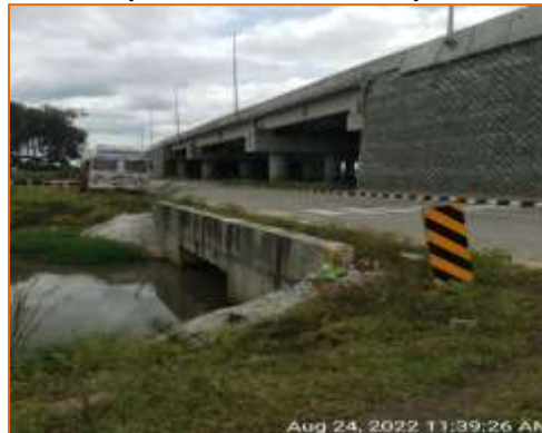
Box culvert at km. 103.850 - RHS (MCW & SR - New Construction)
