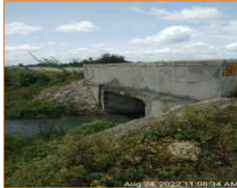
Box culvert at km. 101.823 - RHS (New Construction)
