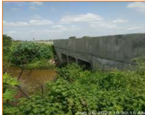
Box culvert at km. 128.229 - LHS (Reconstruction)
