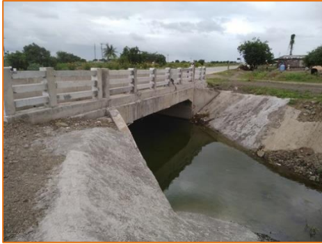
Existing Minor Bridge widening at km. 319.849 on RHS
