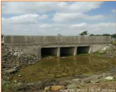
Box culvert at km. 128.229 - RHS (Reconstruction)
