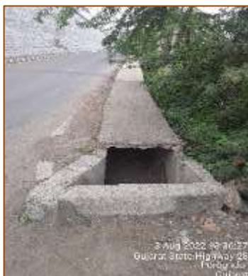
Built-up drain from km. 400+319 to km. 400+700 (LHS)
