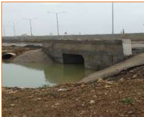
Box culvert at km. 11+950 (LHS)
