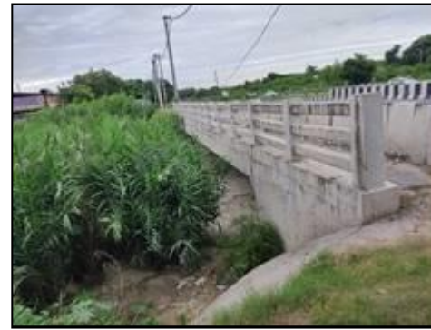
Minor Bridge at km. 75+009 (Structure View)
