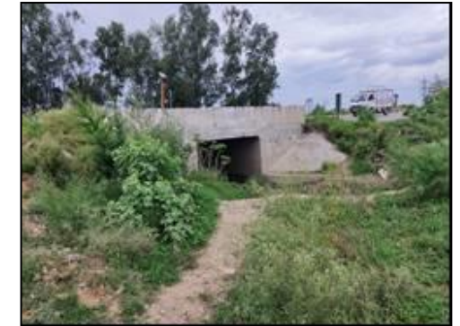
Box Culvert at km. 10+481
