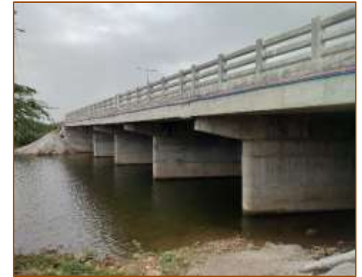
Side View of Minor Bridge at km. 456+533 (LHS) - New
