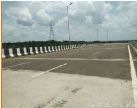
Flyover at km. 106.240 (RHS)
