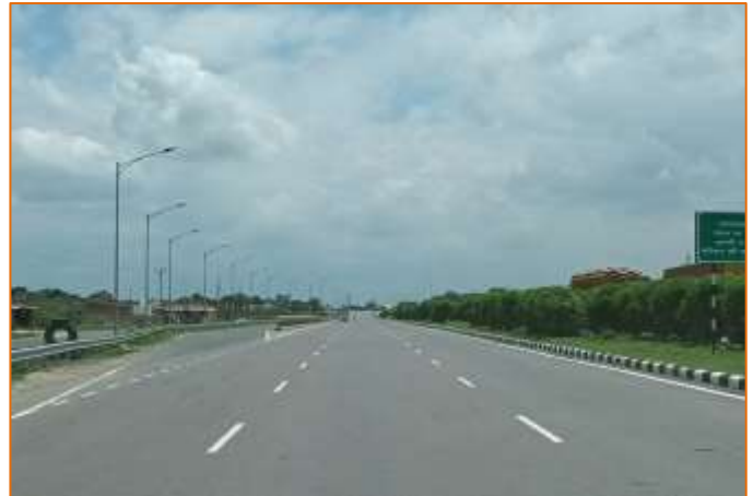
Truck Lay Bye at km. 767+330
