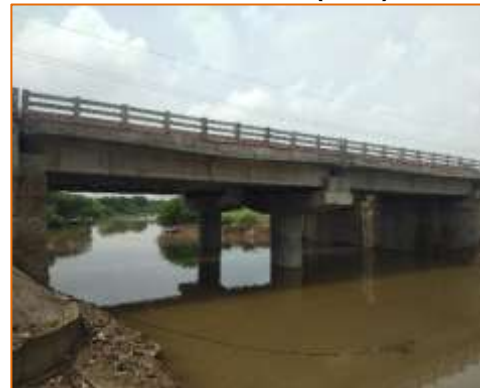
Side View of Minor Bridge at km. 51+730 (LHS)
