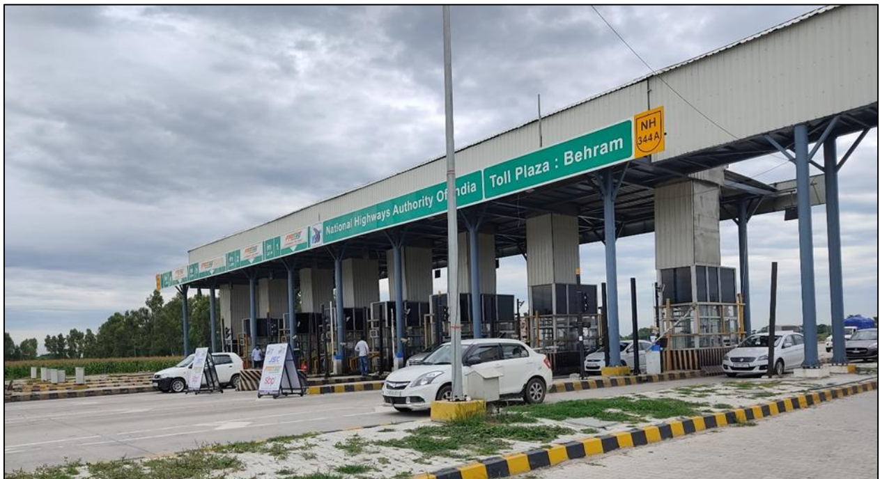
Figure 9-1 View of Behram Toll Plaza (km. 15+300)
