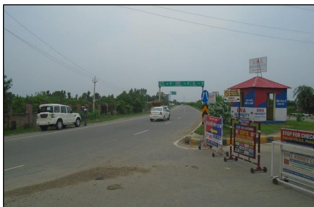
Start of Project Road - Left Carriageway
