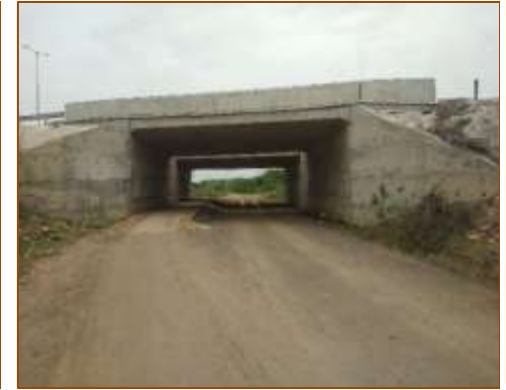
LVUP at km. 488+981 (LHS) - Under COS
