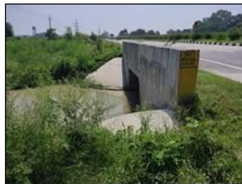
Box Culvert at km. 37+480
