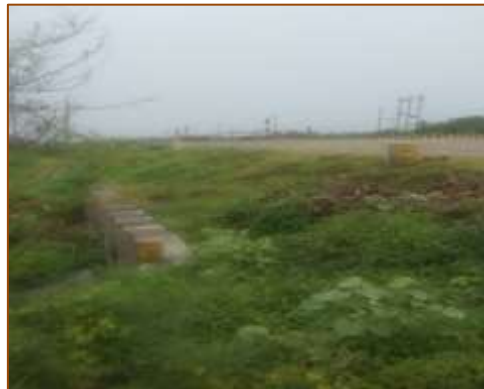
HPC at km. 437+025 (RHS)
