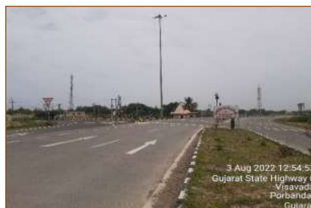
Visawada Bypass at km. 422.800
