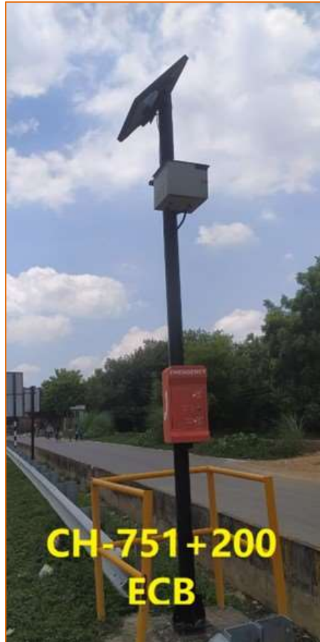
Figure 9-6 ECB at km. 751.200
