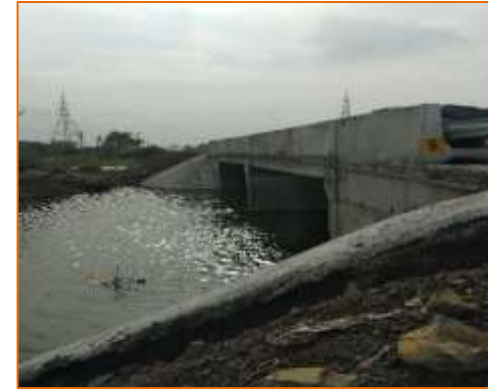
Side View of Minor Bridge at km. 40+807 (RHS)
