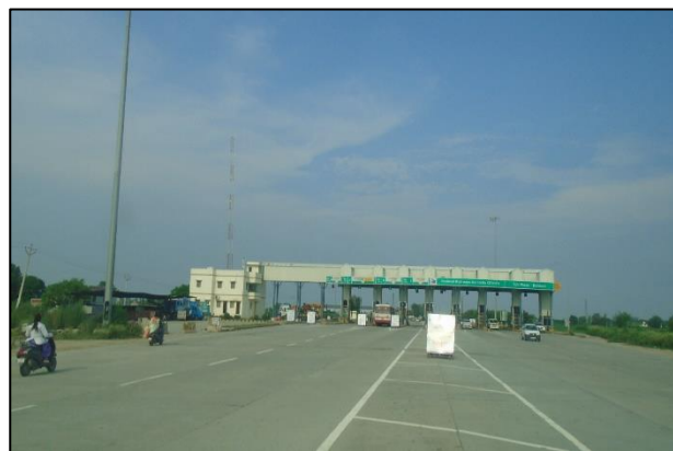
Behram Toll Plaza at km. 15+300
