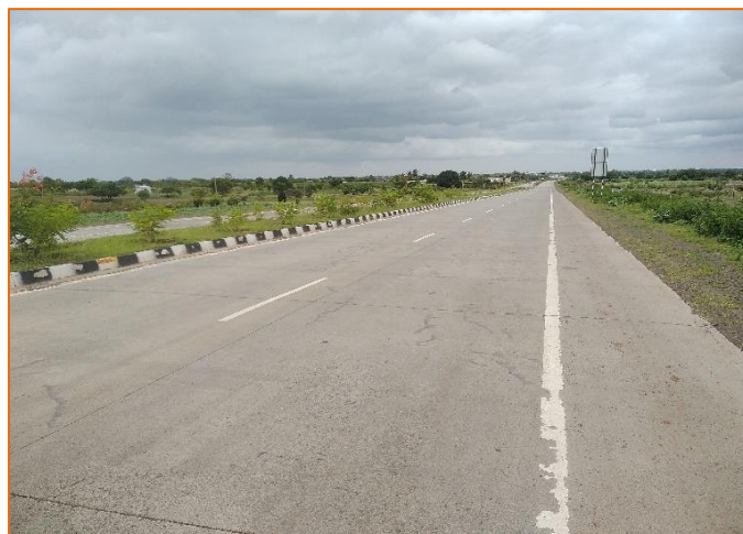
Pavement Condition at km. 319+100 (RHS)
