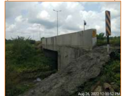
Box culvert at km. 105.290 - LHS (New Construction)
