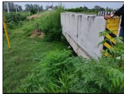
Box Culvert at km. 1+457
