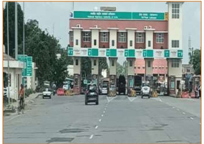
Toll Plaza including Admin Building at km. 747+822
