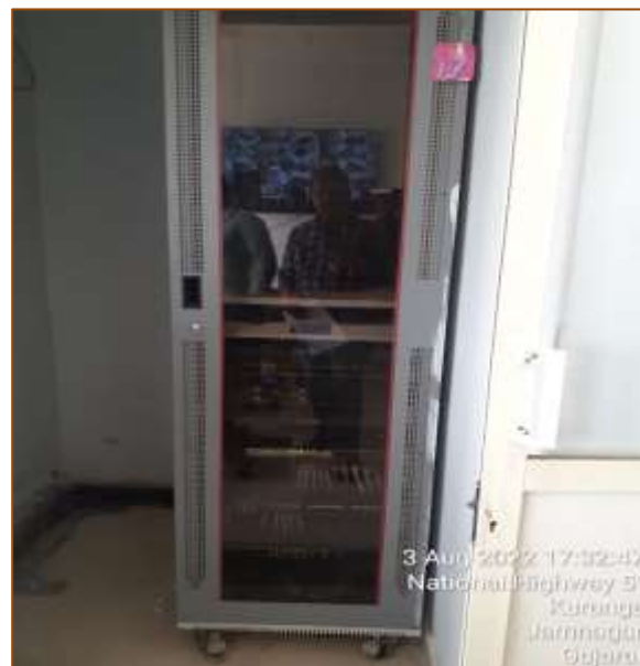
TP-2 at km. 470+875
