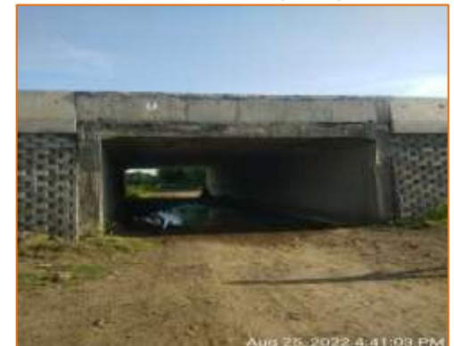
Side View of PUP at km. 104.820 (RHS) - Under COS
