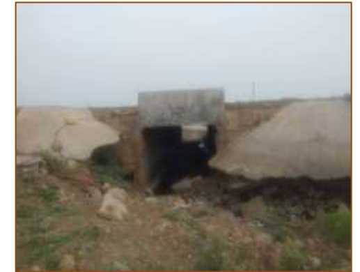
Slab culvert at km. 441+648 (RHS)
