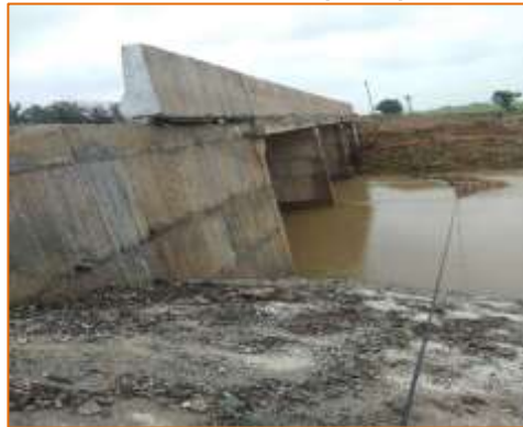
Side View of Minor Bridge at km. 15+270 (LHS)
