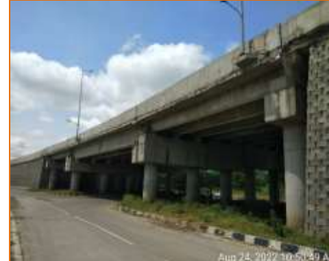
Side View of Flyover at km. 99.900 (RHS)
