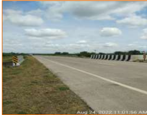
PQC of Minor Bridge at km. 101.260 (LHS)
