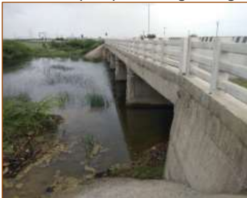
Side View of Minor Bridge at km. 459+038 (LHS) - New
