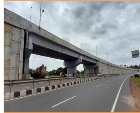
View of UDFO at km. 34+915
