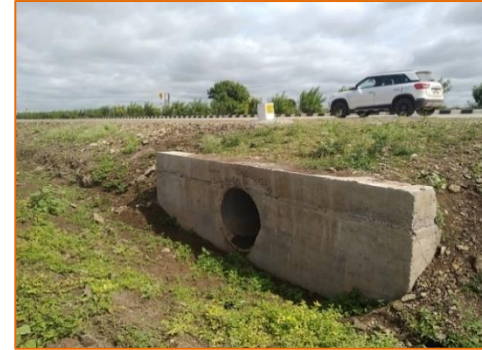
Pipe Culvert at km. 292+135
