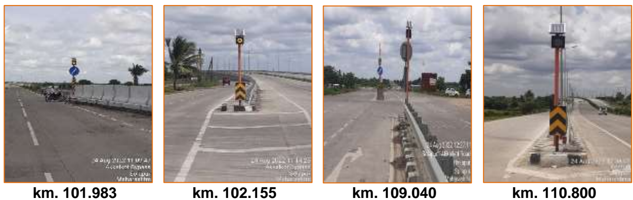
Figure 3-11 Photographs of Highway/Solar Lighting
