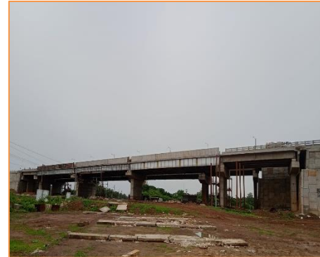
View of ROB at km. 18+677
