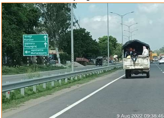
Sign Board at km. 767+100.
