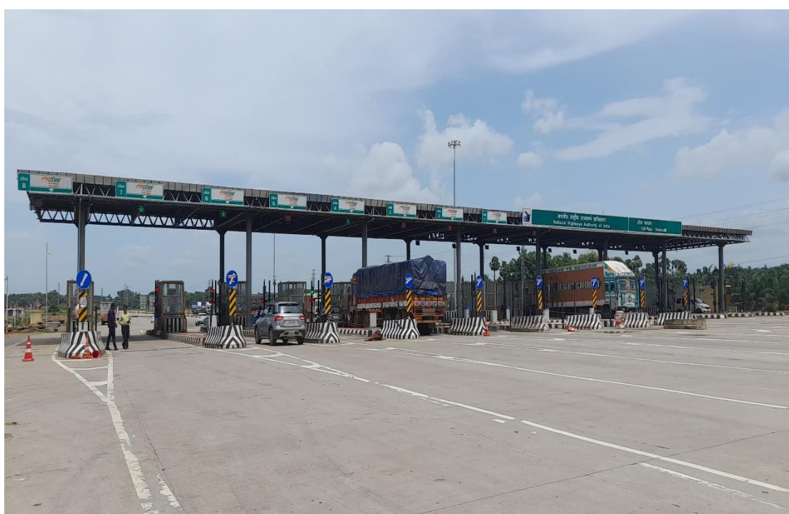
Figure 9-1 View of Toll Plaza (km. 53+700)
