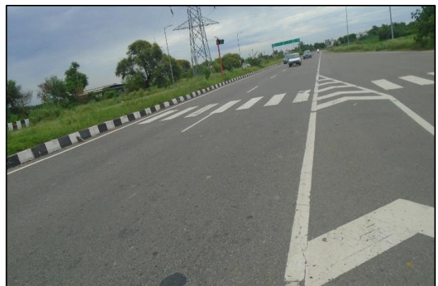
Road Marking at km. 15+800 (RHS)
