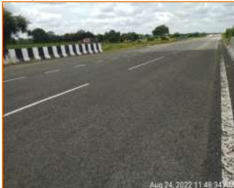
Roughened BC surface of Minor Bridge at km. 104.348 (LHS)
