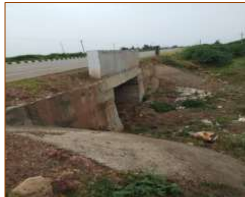
Slab culvert at km. 444+062 (RHS)
