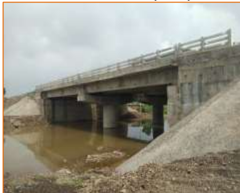
Side View of Minor Bridge at km. 51+730 (RHS)
