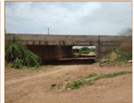
LVUP at km. 488+981 (RHS) - Under COS
