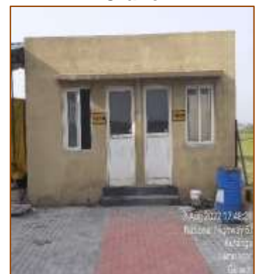
Panel / Pump Room
