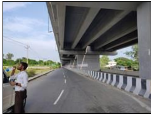
Elevated Structure at km. 25+319
