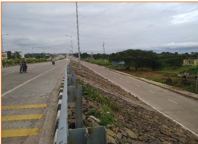
Slope Protection work at km. 284+500.000
