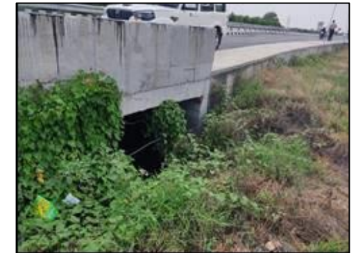
Box Culvert at km. 6+068
