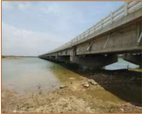
Side View of Major Bridge at km. 422+314 (LHS)
