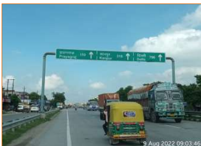
Overhead Gantry Sign at km. 785+040
