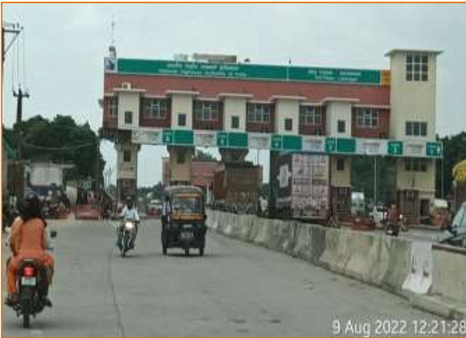
Toll Plaza including Admin Building at km. 747+581
