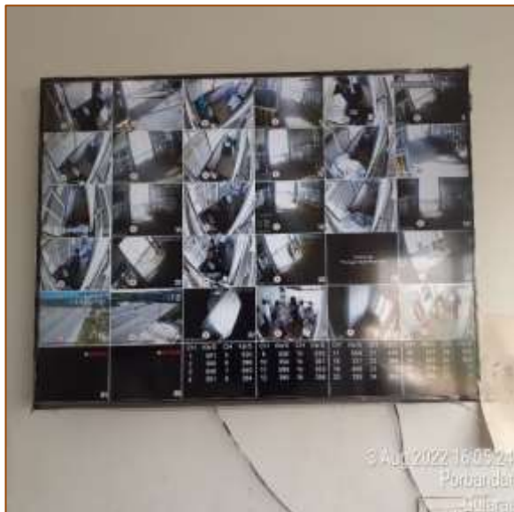
TP-1 at km. 409+500
