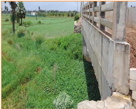
View of Minor Bridge at km. 24+603
