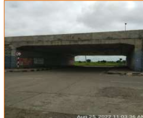
Side View of LVUP at km. 132.025 (LHS)
