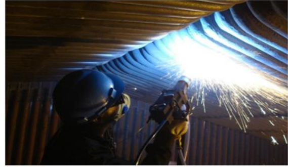
In-Situ ARC spray Coating
