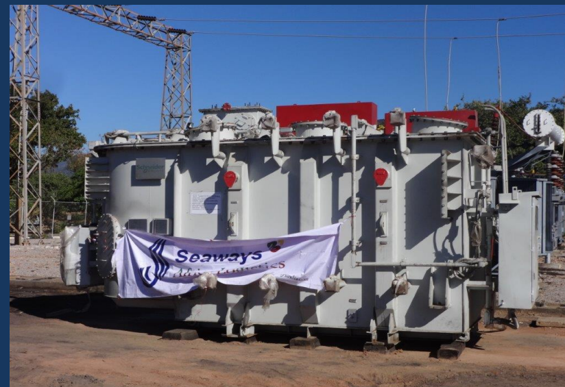
Start-up Power Transformer (20 MVA)
