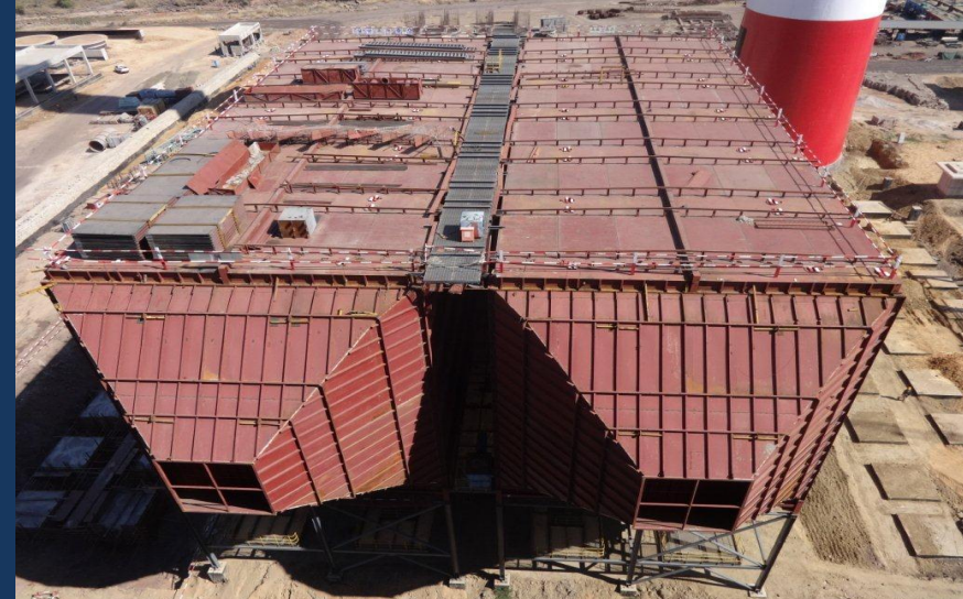
Erection of ESP
