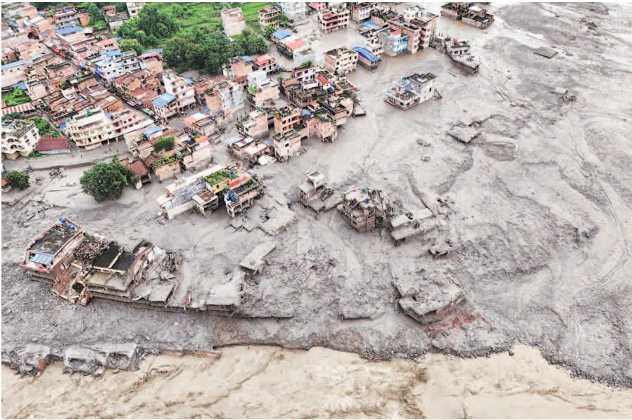
A drone view shows mud covering buildings and property following devastating floods at Trishuli in Nuwakot district, Nepal
