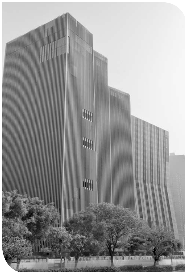
The fins on Max Towers' fascia make it aesthetically distinct and help in energy conservation at the LEED Platinum Green building.
