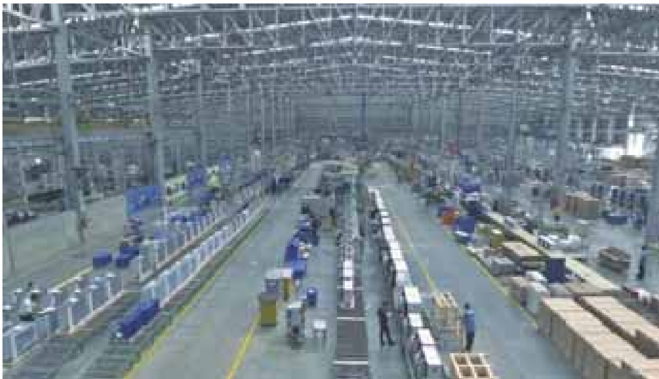
Blue Star's manufacturing facility in Dadra
