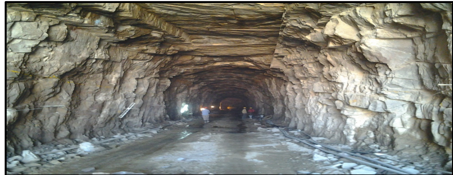
Pranahita - Adit Tunnel-Hard Rock Excavation Completed Stretch
