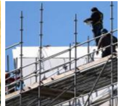
Scaffolding for Construction
