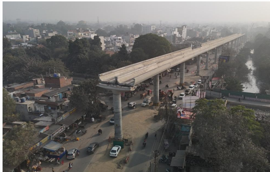
KANPUR METRO construction of 5 elevated stations
