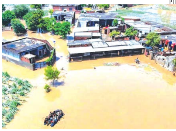
Partially submerged houses at a flood-ravaged area, in Gurdaspur, Punjab
