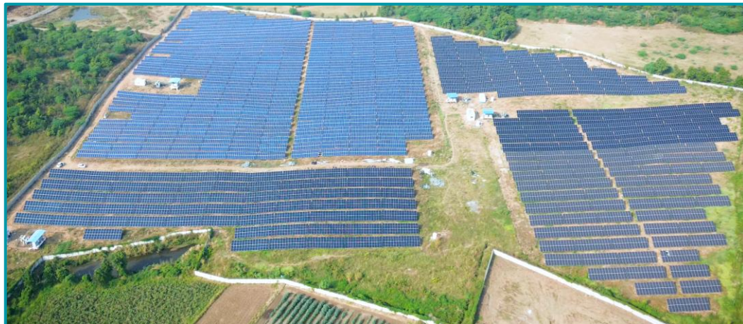
20 MW utility solar for Satyendra Packaging Limited
