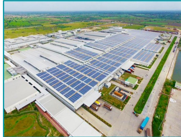
5 MW C&I rooftop for HMSI 1
