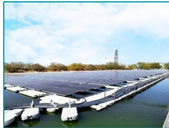
814 KW floating solar for GSFC 2
