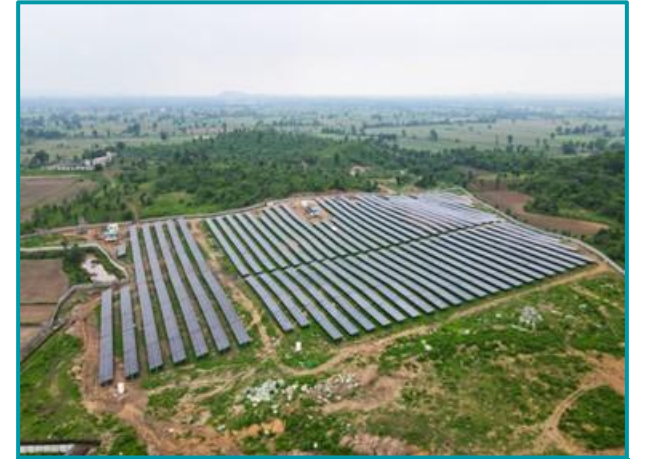
3 MW utility solar for multiple clients
