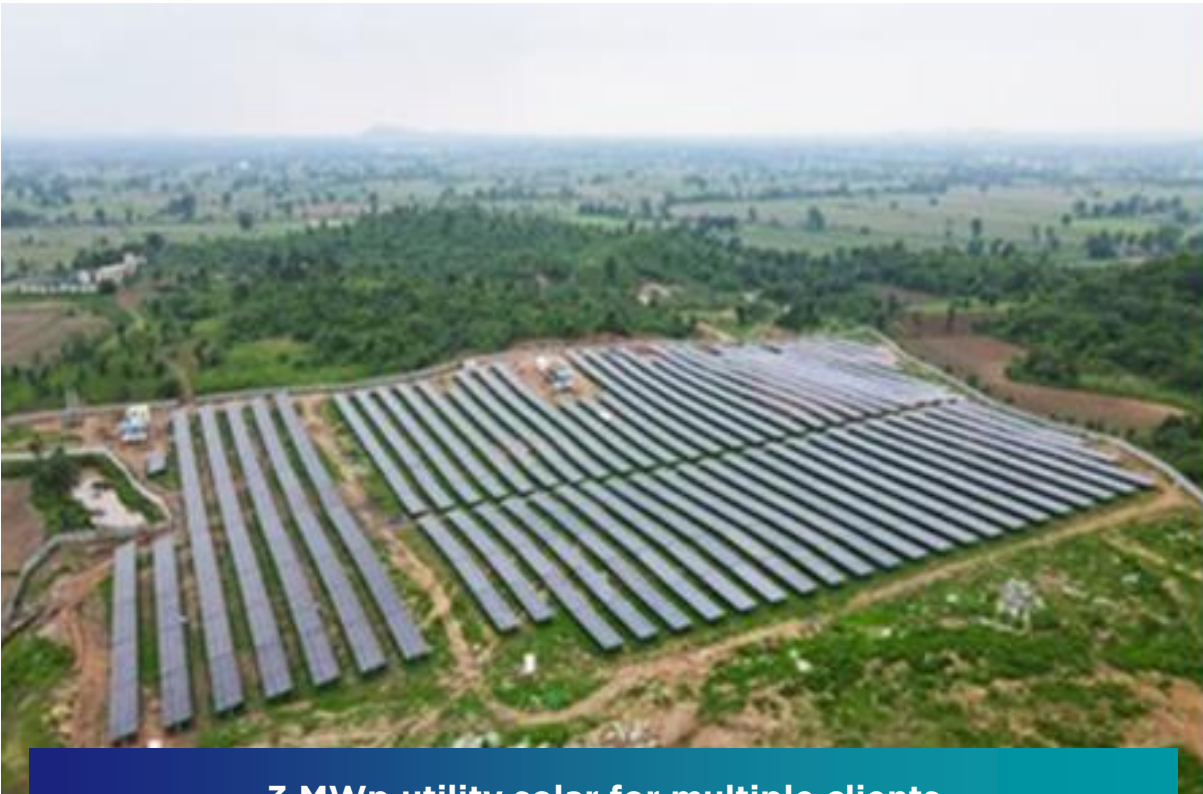
3 MWp utility solar for multiple clients
