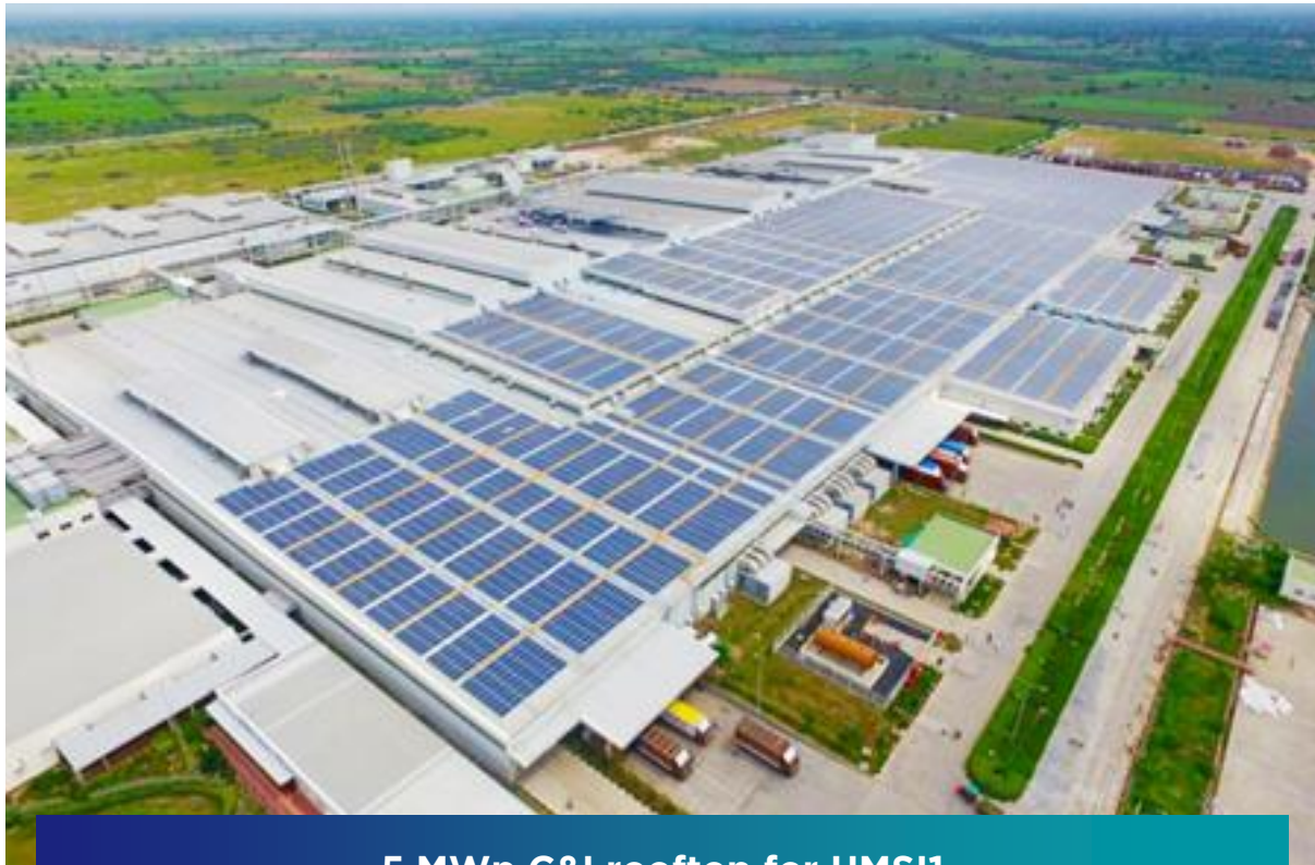
5 MWp C&I rooftop for HMSI1
