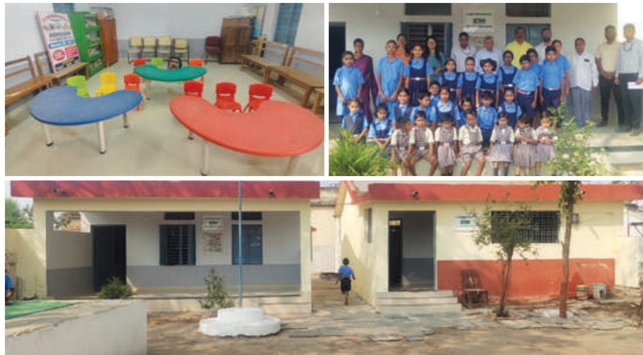
Classroom Renovation - Gat Gram - Panchayat Sawangi (Ghogli), Kalmeshwar, Nagpur
