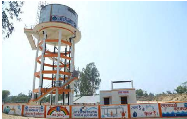
» Rural Water Supply Project under Jal Jeevan Mission, Uttar Pradesh
