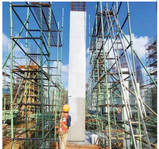
» Acrylic-based curing compound application
