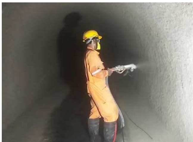
» Rehabilitation of Storm Water Drains by GeoPolymer Technology, Mumbai
