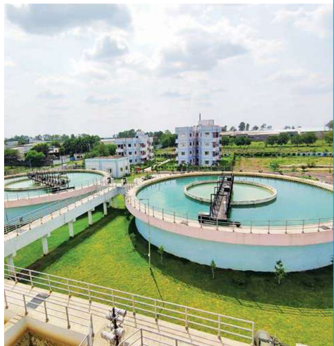
» Dewas Water Project, Madhya Pradesh
