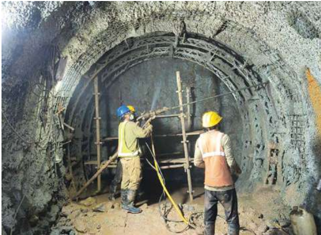
» Priority Sewer Tunnel Phase-I (PST-1) Project, Mumbai
