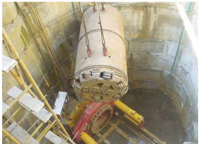
» Microtunnelling Project, Mumbai
