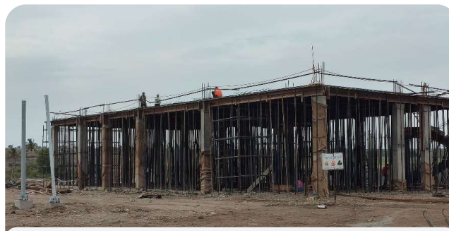
1,000 MWp Solapur, Maharashtra 1
