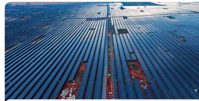
980 MWp Kurnool, Andhra Pradesh 1
