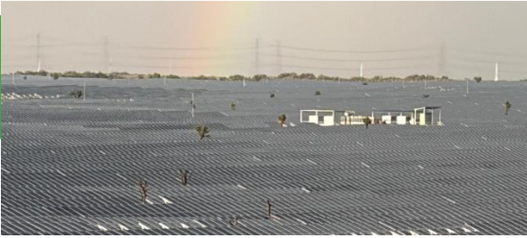
2012 MWp Ground Mounted project at Bikaner, Rajasthan
