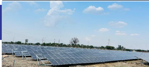
105 MWp Ground Mounted project at Jamnagar, Gujarat
