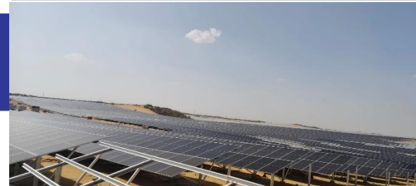
435 MWp Ground Mounted project at Bikaner, Rajasthan
