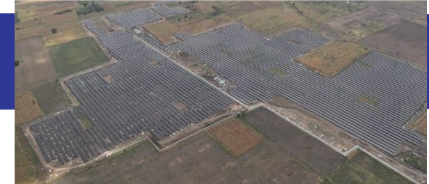
180 MWp Ground Mounted project at Tuticorin, Tamil Nadu
