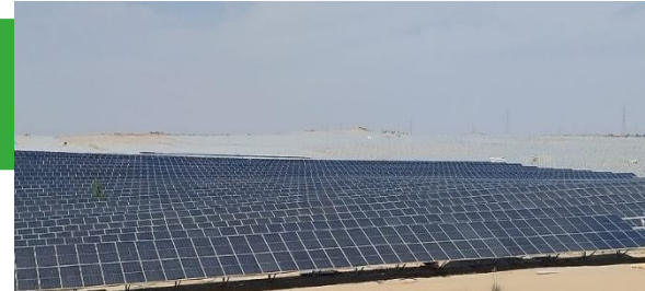
450 MWp Ground Mounted project at Bikaner, Rajasthan
