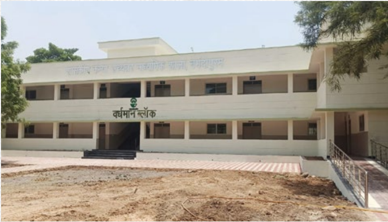
Construction of Government Girls Higher Secondary School Narmadapuram, Budhni, Madhya Pradesh.
