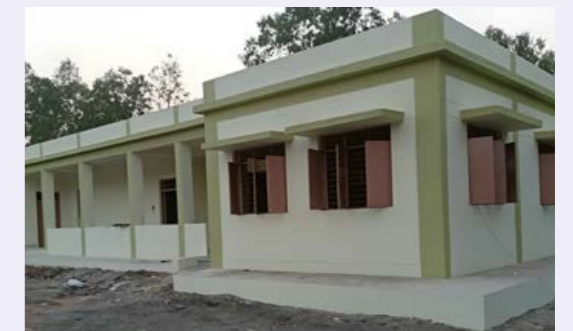
Construction of Government Primary School, Mandheri, Mandideep District, Raisen, M.P.
