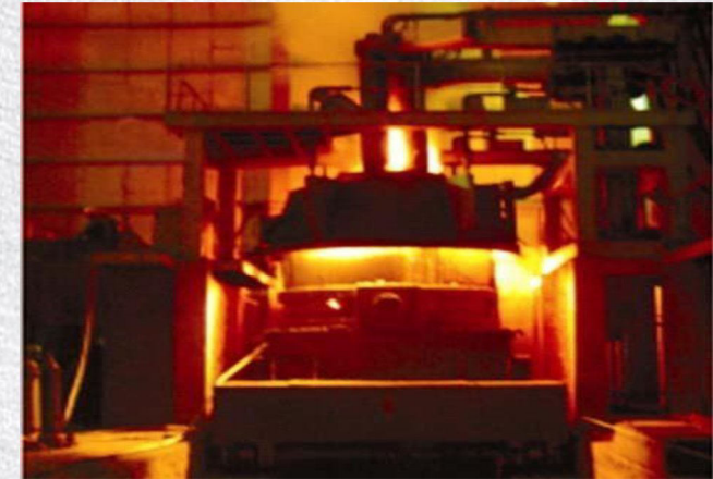
Two Ladle Refining Furnace
