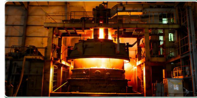
Two Ladle Refining Furnace
