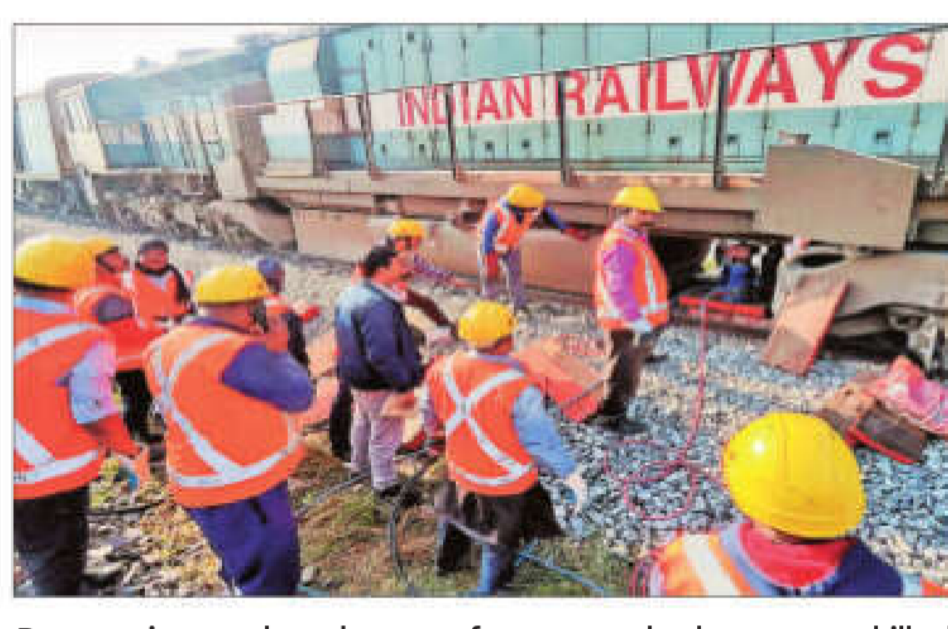
Restoration work underway after seven elephants were killed when the Sairang-New Delhi Rajdhani Express train hit a herd in the Jamunamukh-Kampur section in Hojai on Saturday
