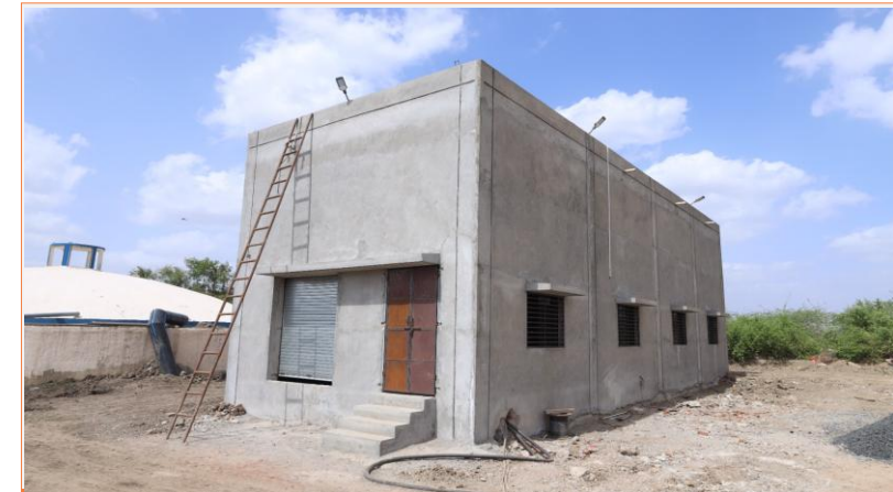
Project Name: GWIL, NC-34 Project Location: Gujarat Value: ₹4.09 Cr
