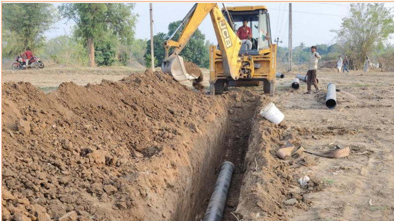
Project Name: Hadaf water Supply Project Location: Gujarat Expected Completion: June 2027
