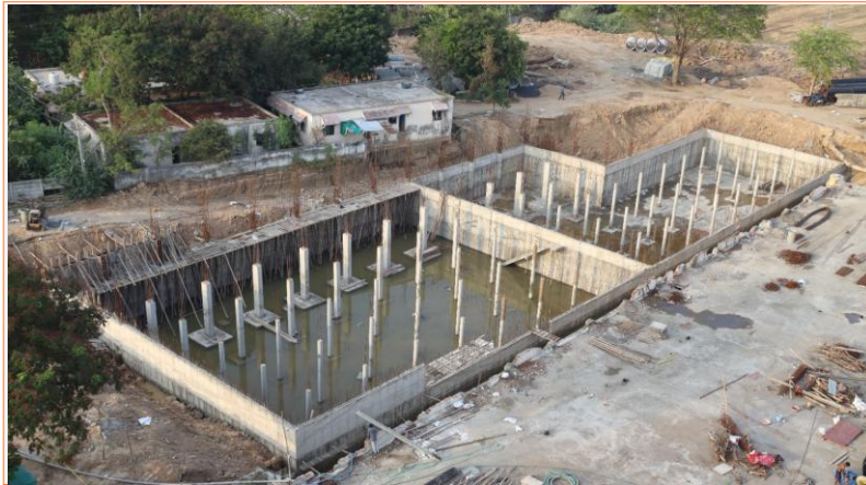
Project Name: Telav Water Supply Project Location: Gujarat Expected Completion: January 2027
