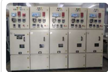
11kV Vacuum Contactor Panel
