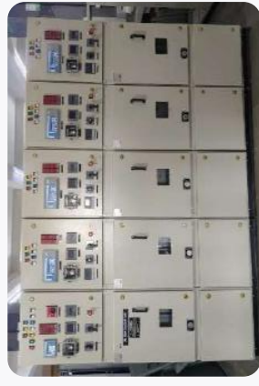
11kV Vacuum Contactor Panel
