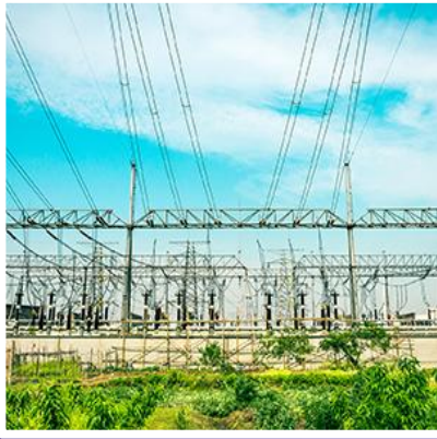
Liasoning With Govt. Authorities And Utilities
