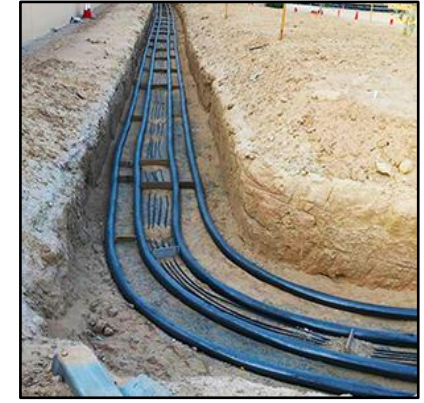
Underground cable laying
