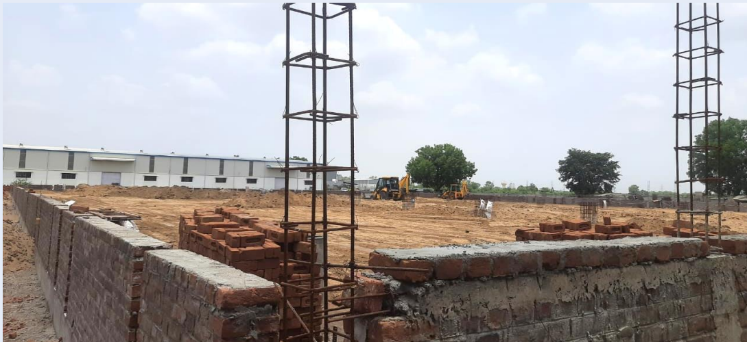
Actual Site Pictures: 419 & 420, khata no. 466 Ganpatpura taluka Karjan, Vadodara, Gujarat
