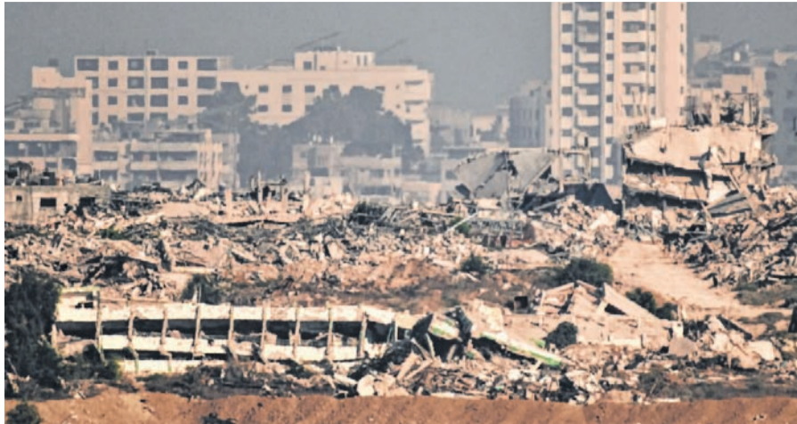
Buildings destroyed during Israeli operations in northern Gaza Strip on Monday
