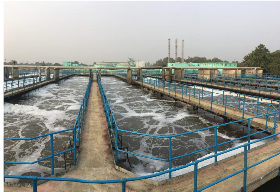
Dinapur Sewage Treatment Plant, Varanasi, UP, India
