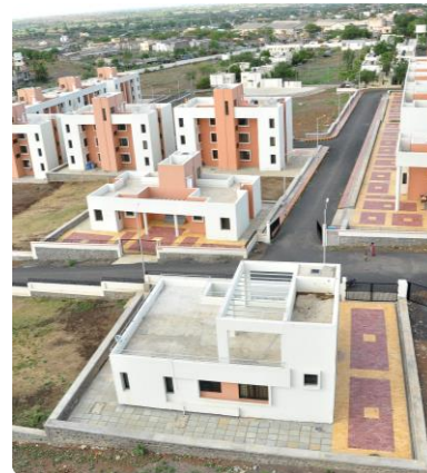
Police Housing Project, Akkalkot
