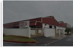
Engineered Metallic Parts Facility (Hobel Bellows)
