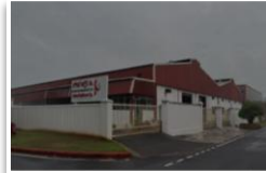
Engineered Metallic Parts Facility (Hobel Bellows)
