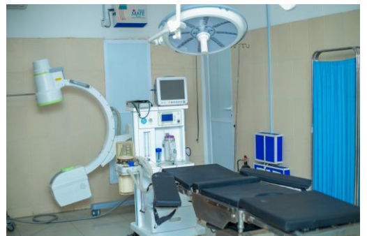
Minor OT Room
