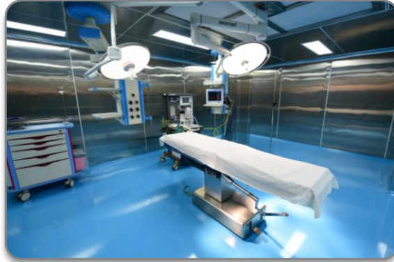
Modular Operation Theater Complex
