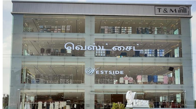
RADIAL ROAD, CHENNAI
