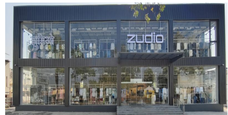
SHAKUNTALA COMPLEX, SHIRPUR
