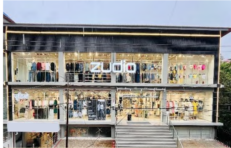
MAXON TOWER, PALAMPUR
