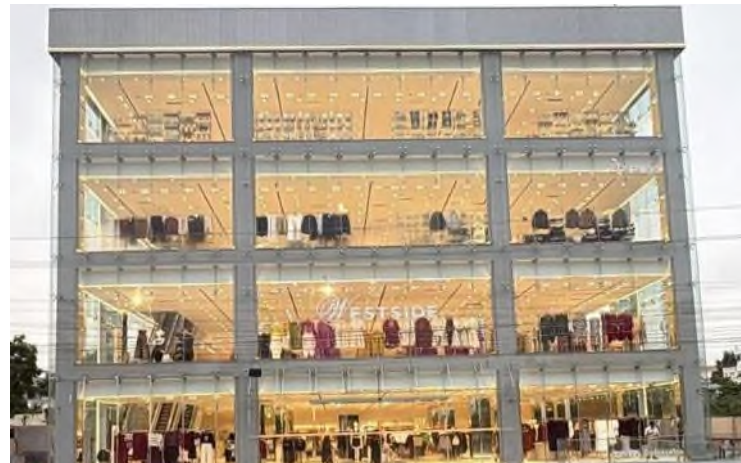
SNB Tower, Udaipur
