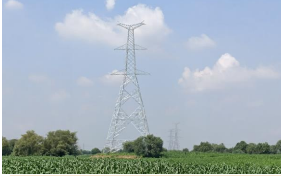
Koppal-II PS – Narendra 765 kV D/C line, Karnataka
