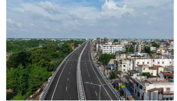
Begusarai elevated road project, Bihar
