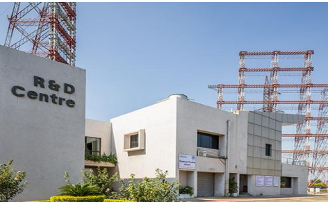
Tower Testing Facility - Deoli
