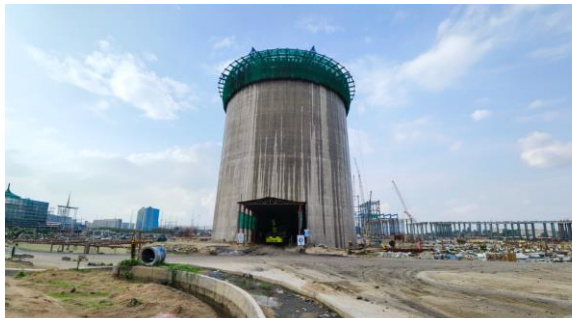
275 m tall Twin Flue RCC chimney, Koderma (KTPS) Phase-II, Jharkhand
