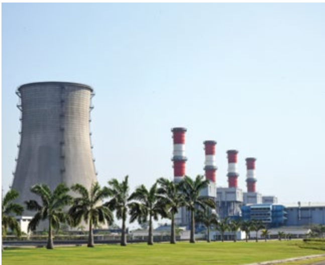
SUGEN Power Plant
