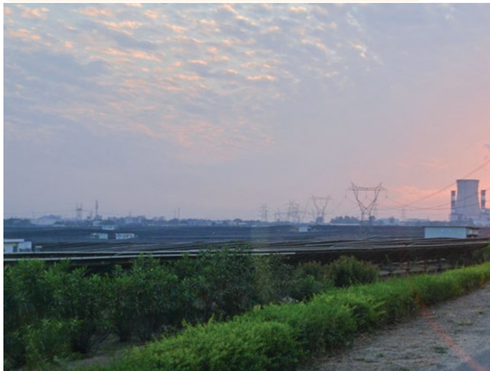
Transmission Tower, Surat
