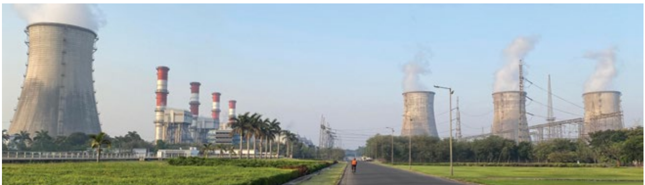
1,530 MW Gas-based SUGEN & UNOSUGEN Power Plants, Surat
