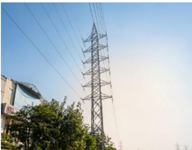
Transmission Tower, Ahmedabad
