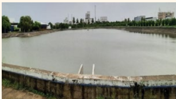
Rain Water Harvesting System at DGEN
