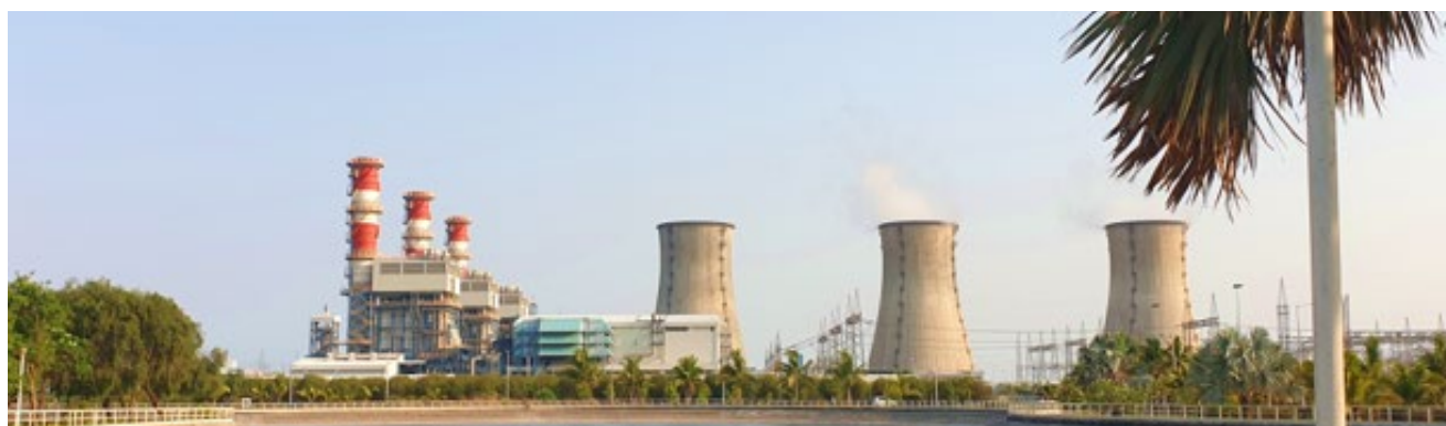
SUGEN Power Plant
