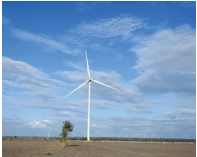
60 MW Wind Power Plant, Karnataka
