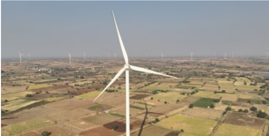
126 MW Wind Power Plant, Maharashtra
