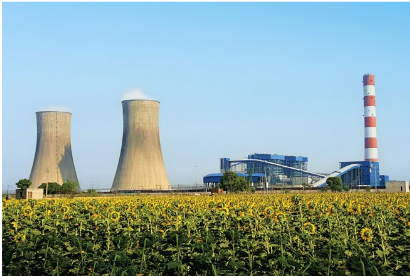
1400 MW Coal based NABHA Power Plant, Punjab
