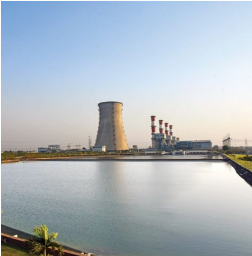
Rain water collection pond at SUGEN
