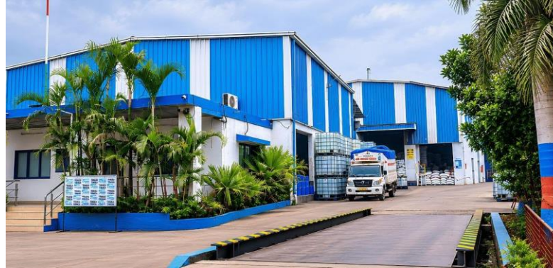
02 Wada, Maharashtra Tyre Recycling Plant
