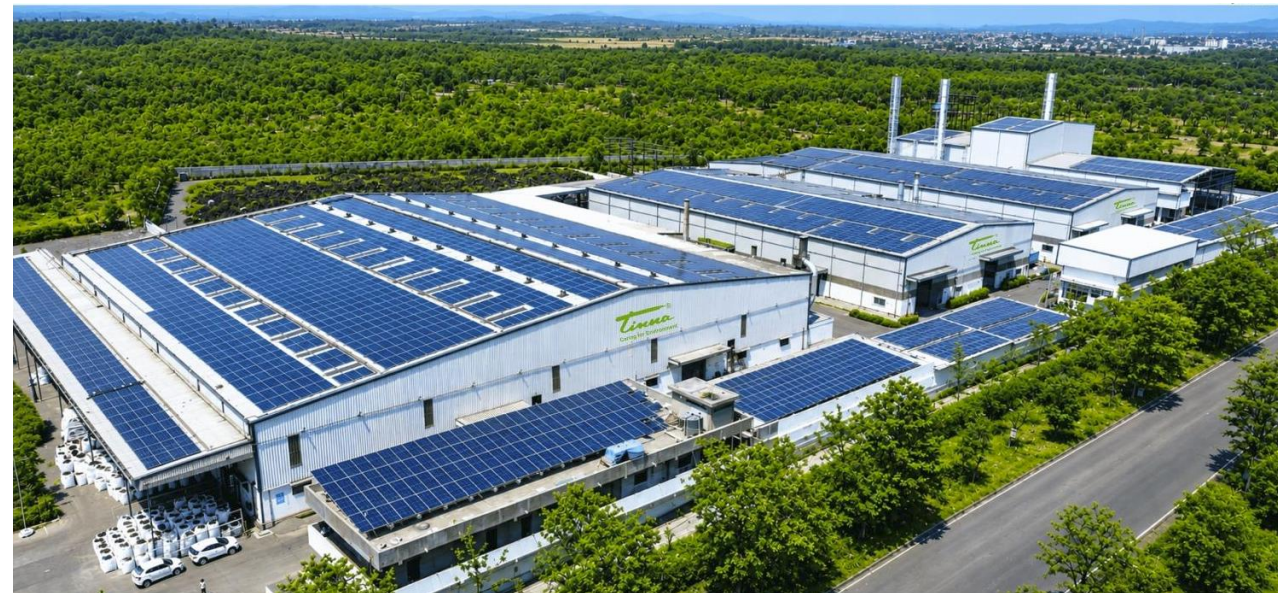
Fully Integrated Tyre Recycling Complex with Rooftop Solar at Varale (Maharashtra)
