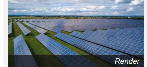
Solar Plant installation delivering long term cost saving
